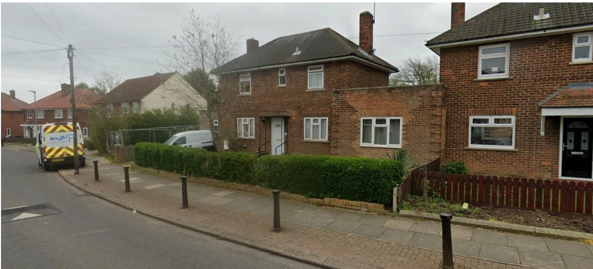
47 Coleridge Gardens, Darlington from the south west
