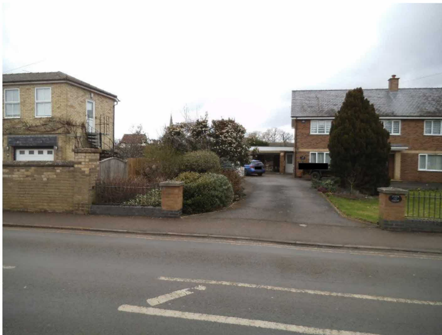
Existing access and wall.
