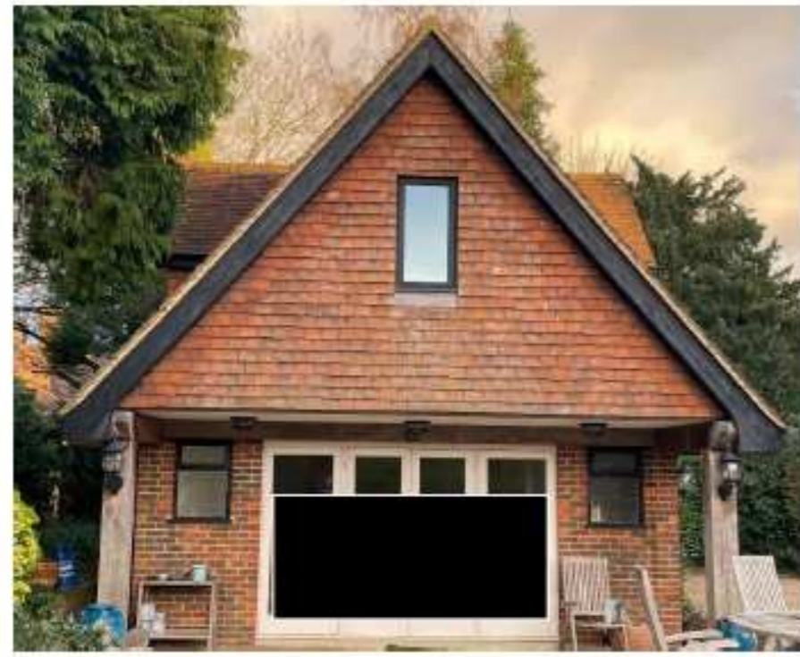
3 Photos of the Swallow tiles & brickwork design proposed, on another completed project.
