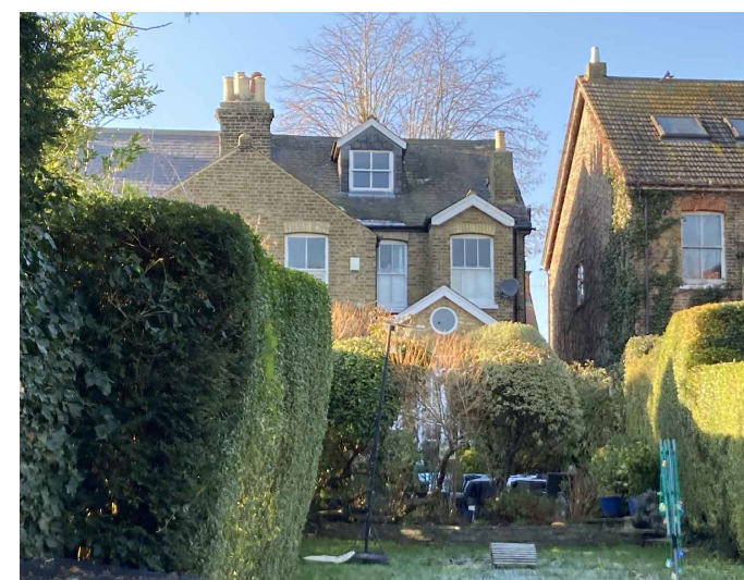
Photo 3: Existing rear elevation from garden
