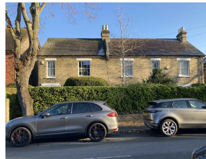
Photo 1: Existing front elevation
