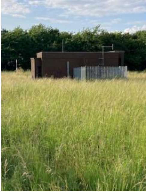
Figure 9. View of substation building from south.
