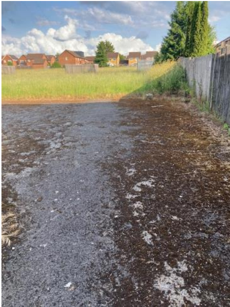
Figure 5. Tarmac access track in north western corner of site.
