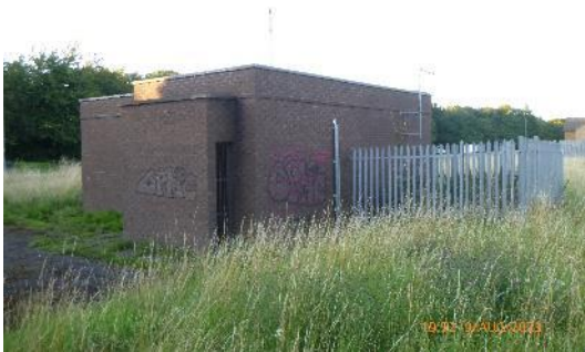
Figure 1. Substation building (image facing north east).
