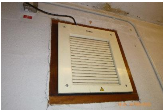
Figure 5. Internal view of vent on eastern elevation (sealed).
