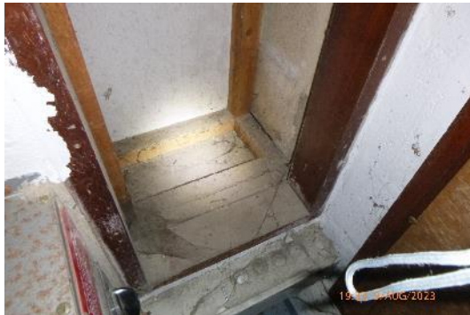
Figure 7. Interior in good condition.
