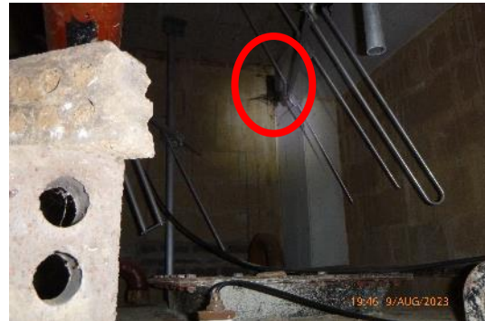
Figure 8. Hole in wall suggests cavity walls are present.
