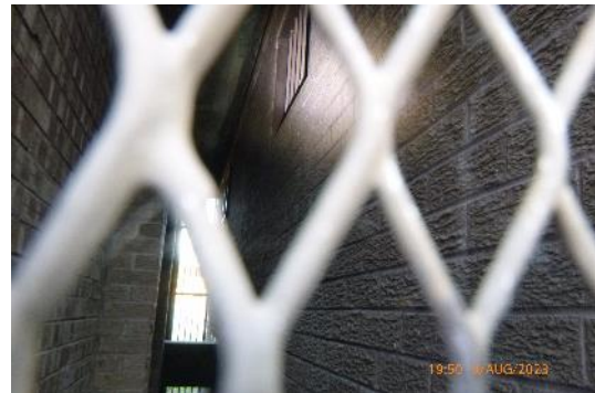
Figure 4. External view of vents on eastern elevation.
