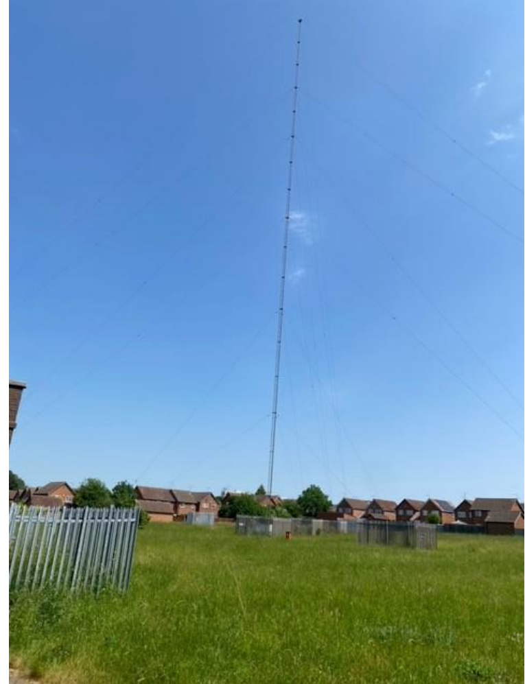
Existing mast (now removed) looking South East. Photo taken in north west corner of site
