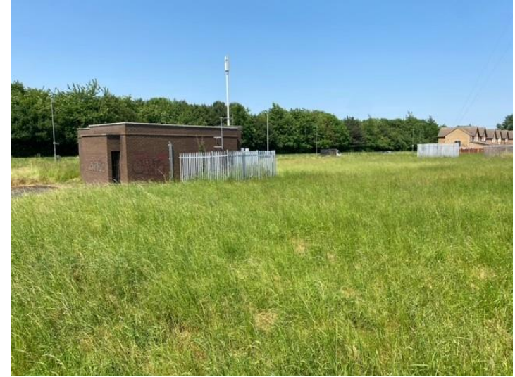
Looking north at the single storey brick service building to be demolished
