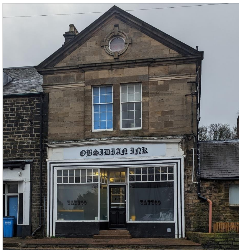
Plate 41. View south at Grade II Listed shop from Front Street
