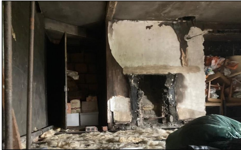
Plate 31. View west towards second floor fireplace
