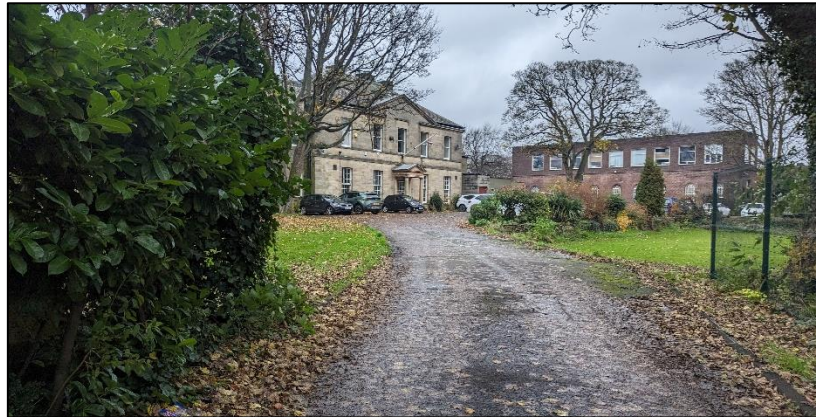
Plate 15. View northeast across site
