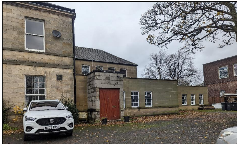
Plate 19. View northeast at the eastern wing
