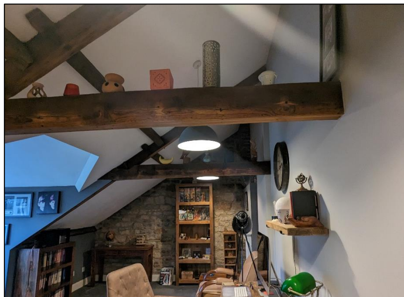
Plate 34. View west across attic space
