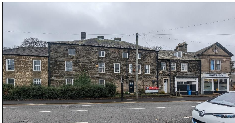
Plate 20. View south at the rear elevation from the Black Bull carpark
