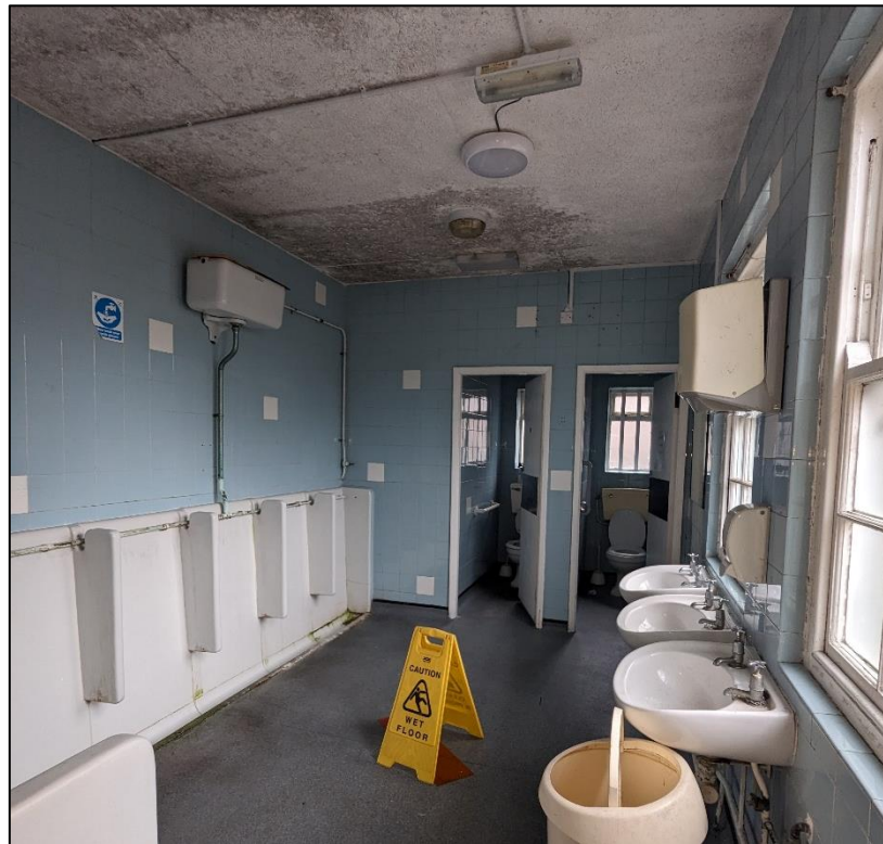
Plate 23. Toilet block in eastern wing
