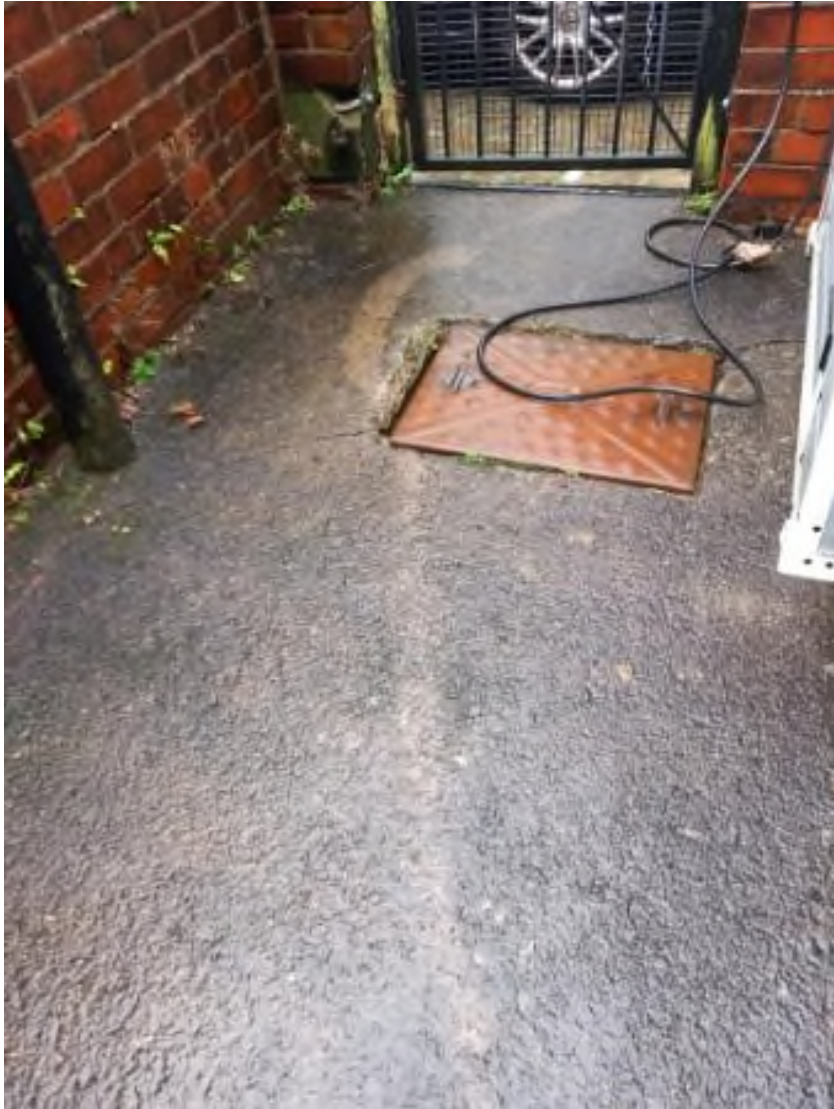
Photograph No 5: View of Concrete Surfacing in Rear Yard
