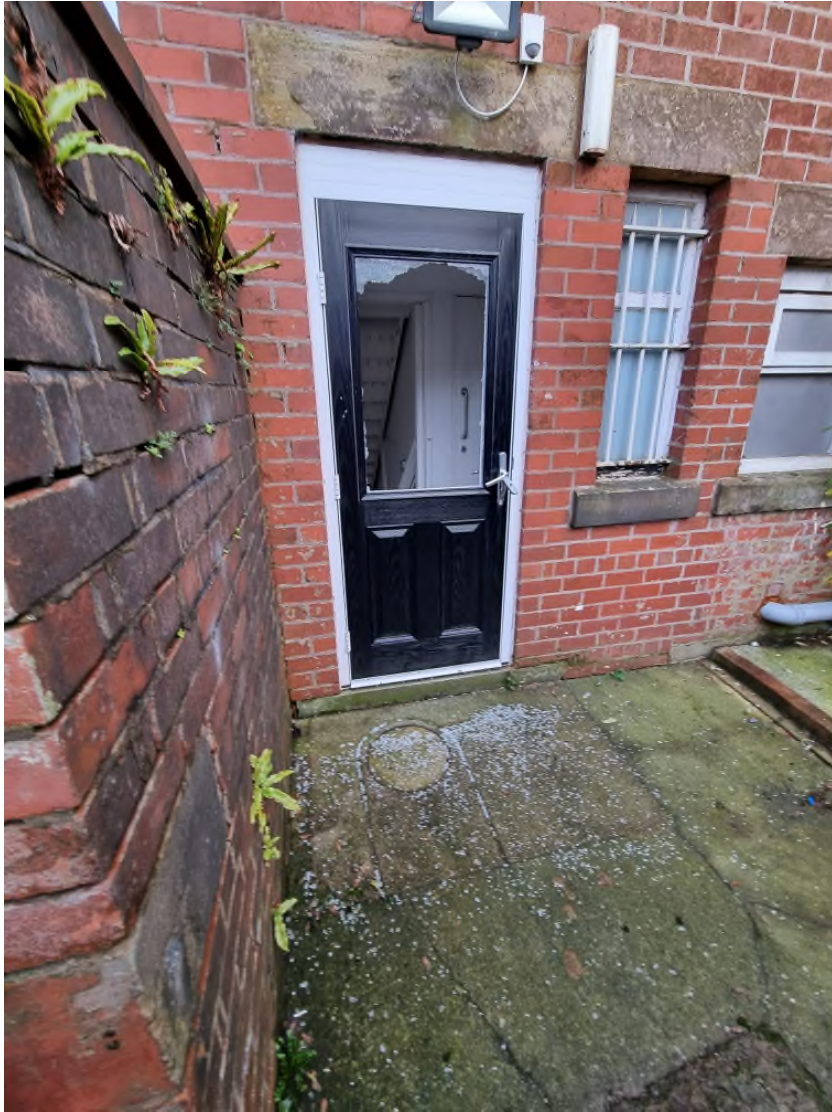
Photograph No 7: View of Concrete Surfacing in Rear Yard
