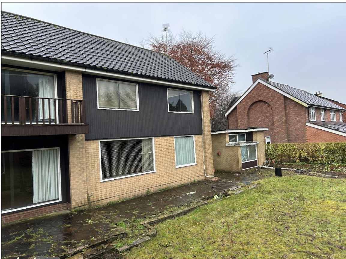
Plate 8 – Southern aspect of the structure on site
