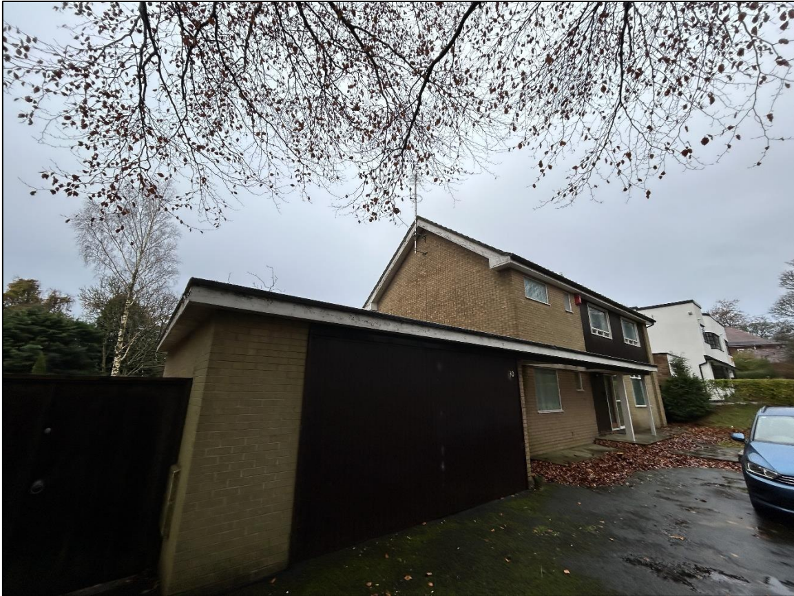
Plate 11 – Eastern elevation of the building
