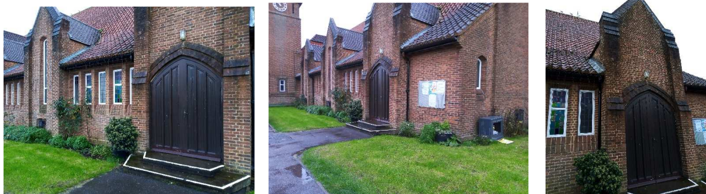
Photos above show the existing steps which are a barrier to independent access.
