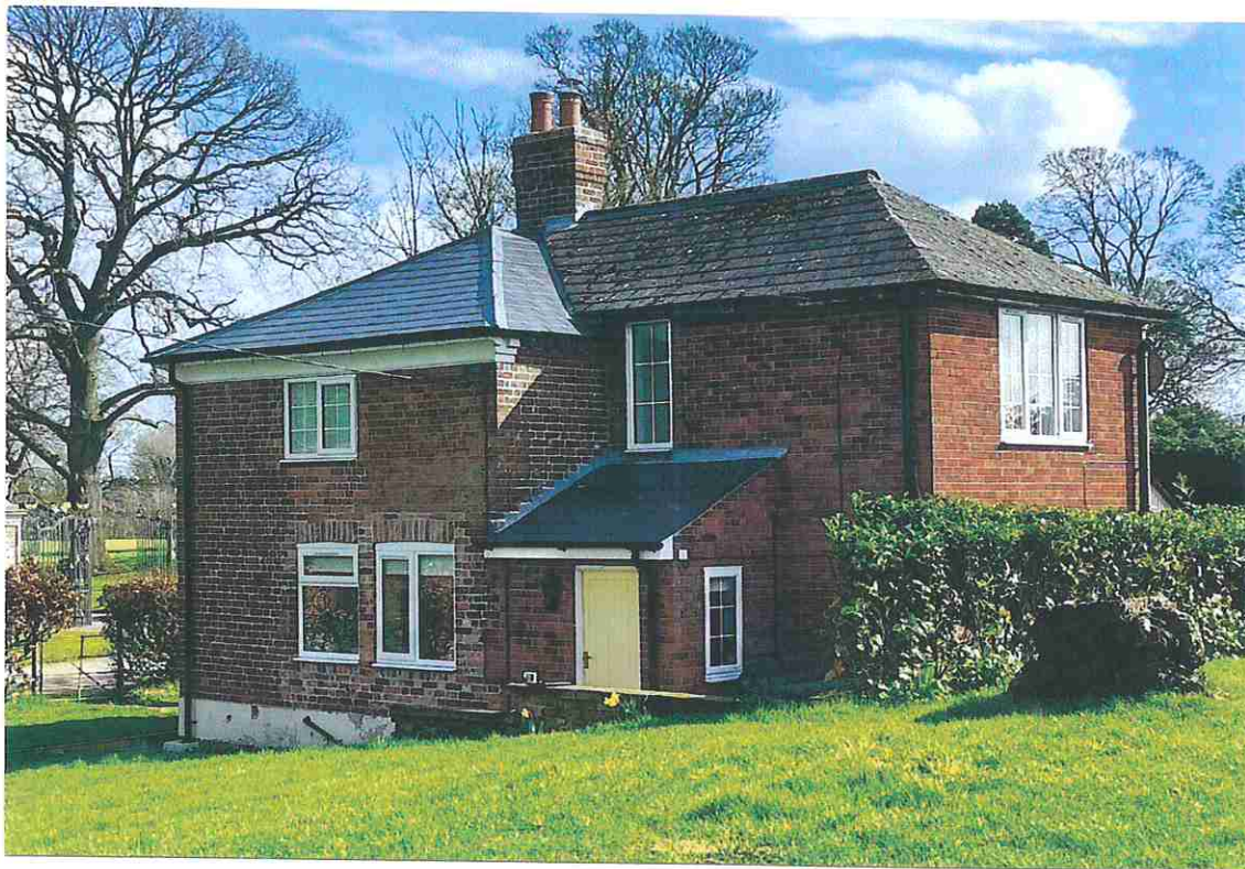
PHOTOGRAPH 11 - GENERAL VIEW OF THE HOUSE FROM WITHIN THE GARDEN WHICH SHOWS HOW THE EARLIER EXTENSION HAS A HIGHER EAVES AND RIDGE THAN THE ORIGINAL HOUSE.
