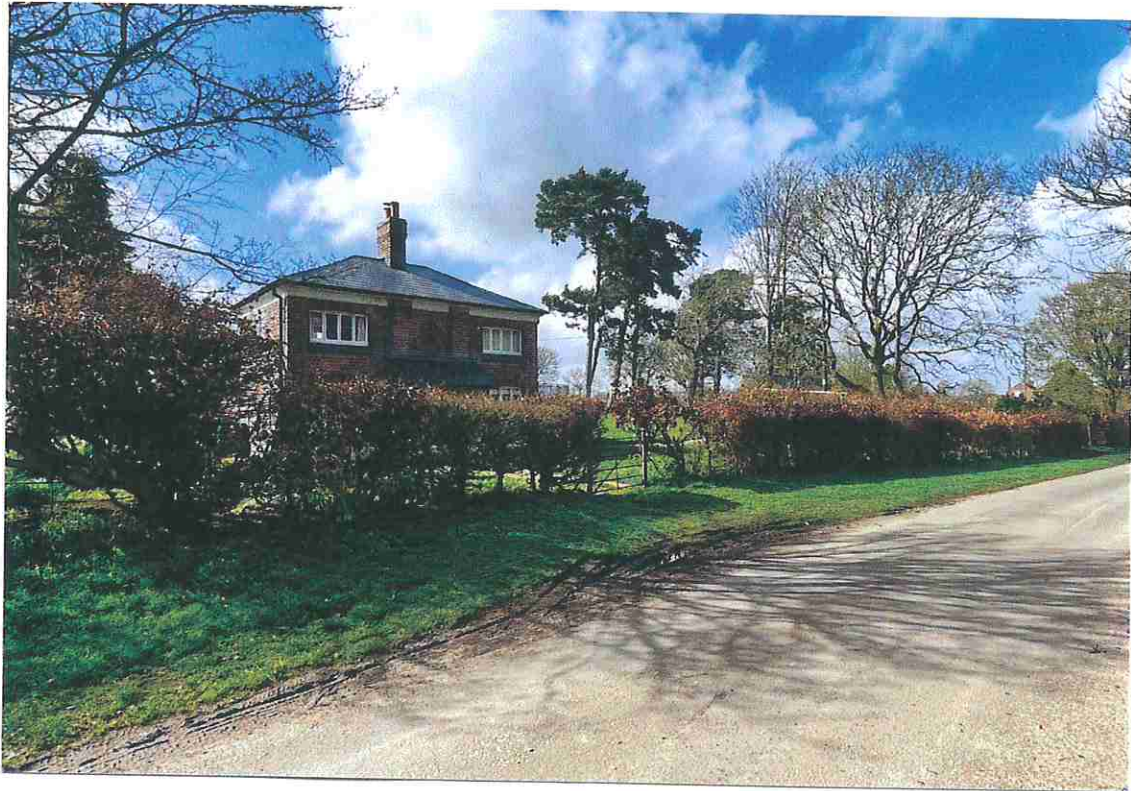
PHOTOGRAPH 4 - GENERAL VIEW FROM THE ACCESS TO PEPLOW HALL LOOKING BACK TOWARDS LODGE COTTAGE.
