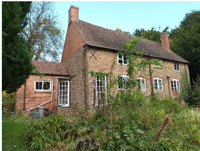
View of the cottage and the 1950's extension to be demolished.
