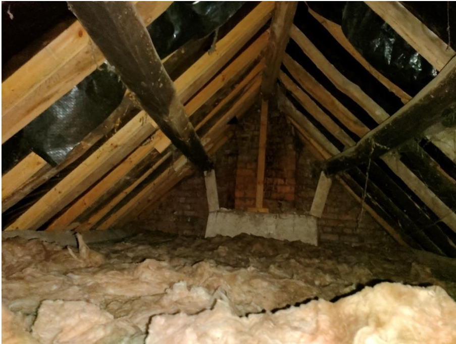
Plate 7: Roof void, towards western end.
