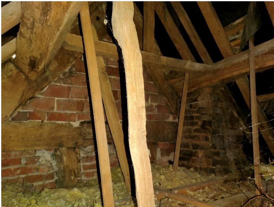
Plate 6: Roof void, towards eastern end.
