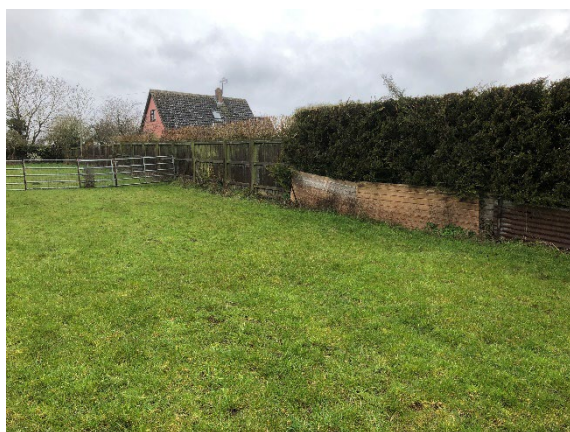
Managed conifer hedge and closed board fence along the north-east boundary.
