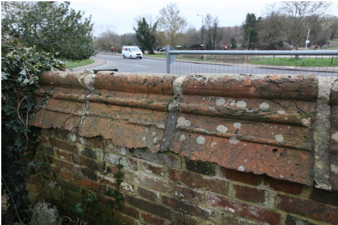
Illus. 24. A detail of the finely moulded re-used coping tiles above the recently rebuilt section of the roadside wall seen from the garden of no. 12 to the east (hidden behind the green portable shed in illustration 22).
