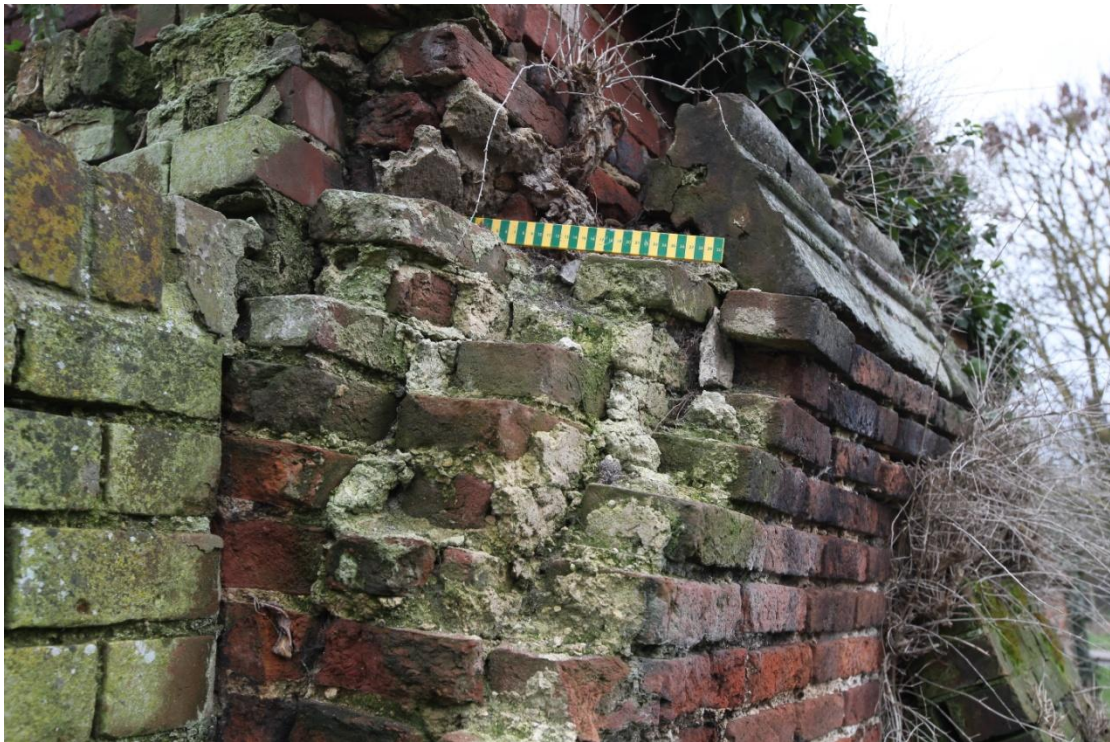
Illus. 18. A detail of the recently damaged corner of the 16 th or 17 th century wall in illustration 17 (1), showing its width of 14 inches or 35 cms.
