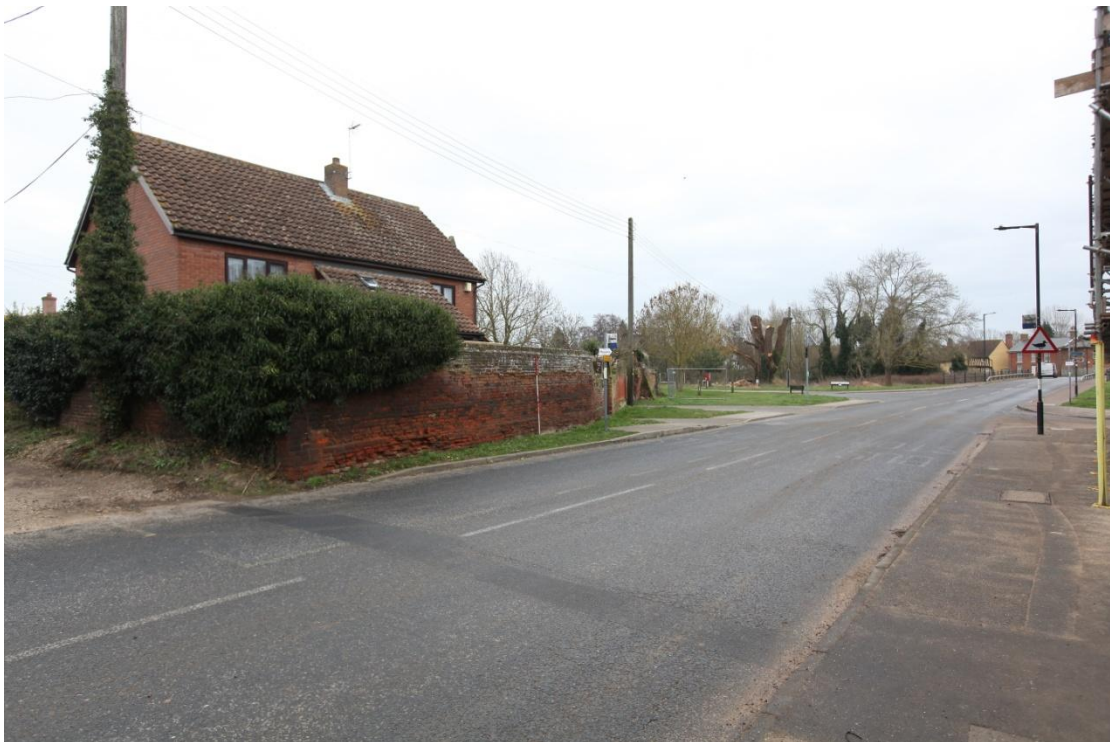
Illus. 6. Bridge Street from the north showing the marked change in angle of the farm yard wall that now belongs to River View. The demolished barn adjoined the field track on the left known today as Sun Court Gardens.
