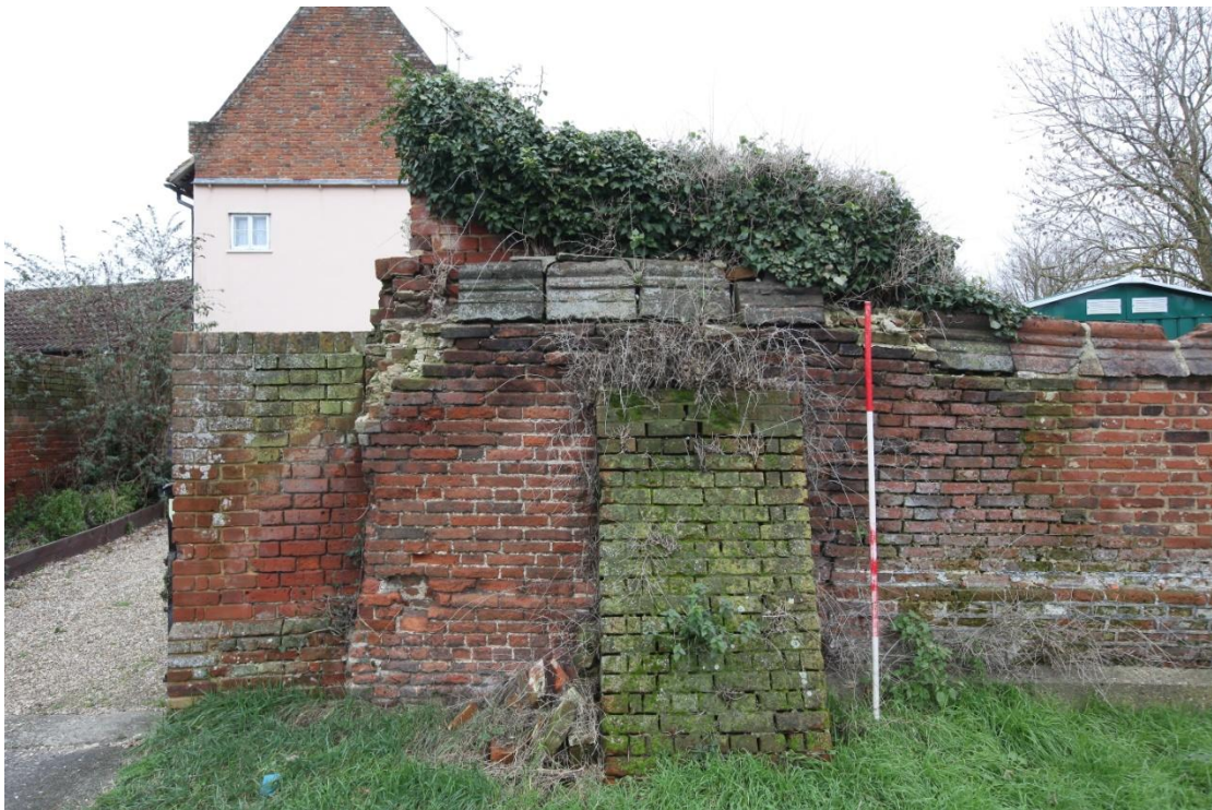
Illus. 12. The large 19 th century buttress (3) pre-dates the overgrown 20 th century brick garden shed which overtops the wall at this point. The coping tiles probably indicate the wall's original height of 8 ft or 1.2 m, which is taller by three courses than the rebuilt section (5) to the right.
