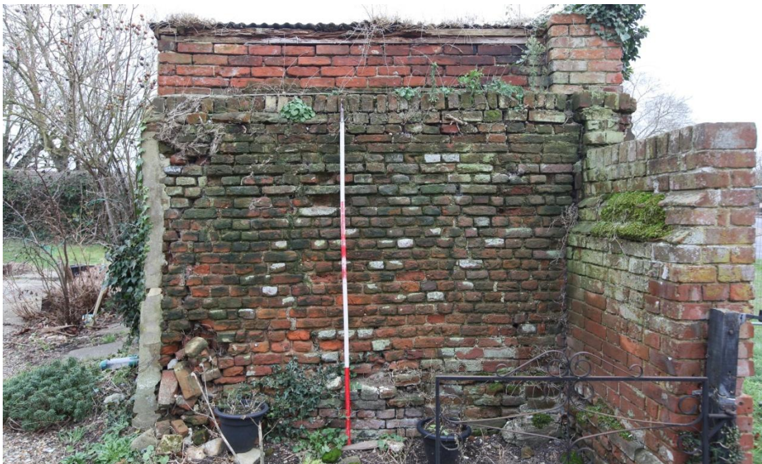
Illus. 20. The former northern wall of the 19 th century garden to the south of the house (8), as seen from the entrance to no. 12 to the north. The left-hand edge is formed by broken bricks and this wall once continued to the south-western corner of the house (connecting to the fragment that still remained in 1962 as shown in figure 10). It is crudely constructed almost entirely of headers and is overtopped by the lighter and more uniform bricks of the mid-20 th century garden shed which terminates to the right in a recent pier built directly upon the oldest part of the wall.
