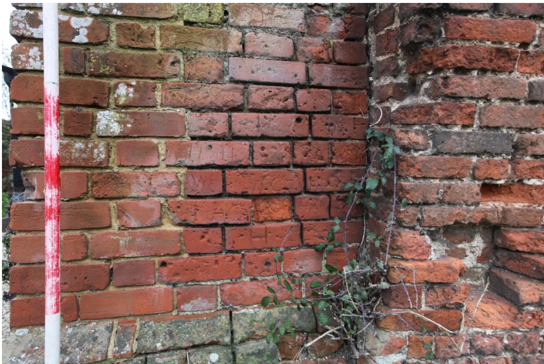
Illus. 16. The short section adjoining the present entrance to the left (4) consists of uniform soft reds of 2.5 inches by 9 in the typical manner of the 19 th century. It bears a surprising number of incised initials that would have been impossible on the harder 17 th century bricks to the right. The left-hand half of this section has been recently built with matching bricks as indicated by their lighter colour and cement mortar.
