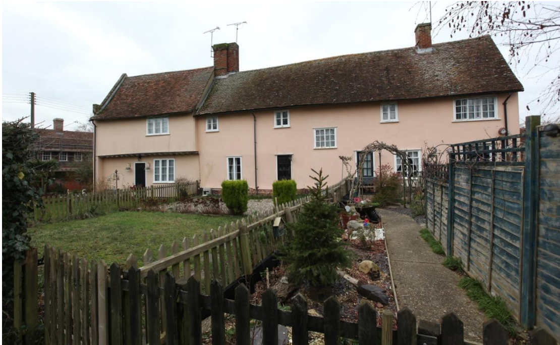
Illus. 3. The southern facade of the house, with nos. 14 and 16 to the right and the taller jettied range of no. 12 on the left. The gardens are now divided by fences but were formerly a single, larger garden separated by the brick boundary wall from the waste ground against the road. No. 12 was built either as the rear wing of a demolished house on the street to the left or as the new parlour of an older and lower house on the right.
