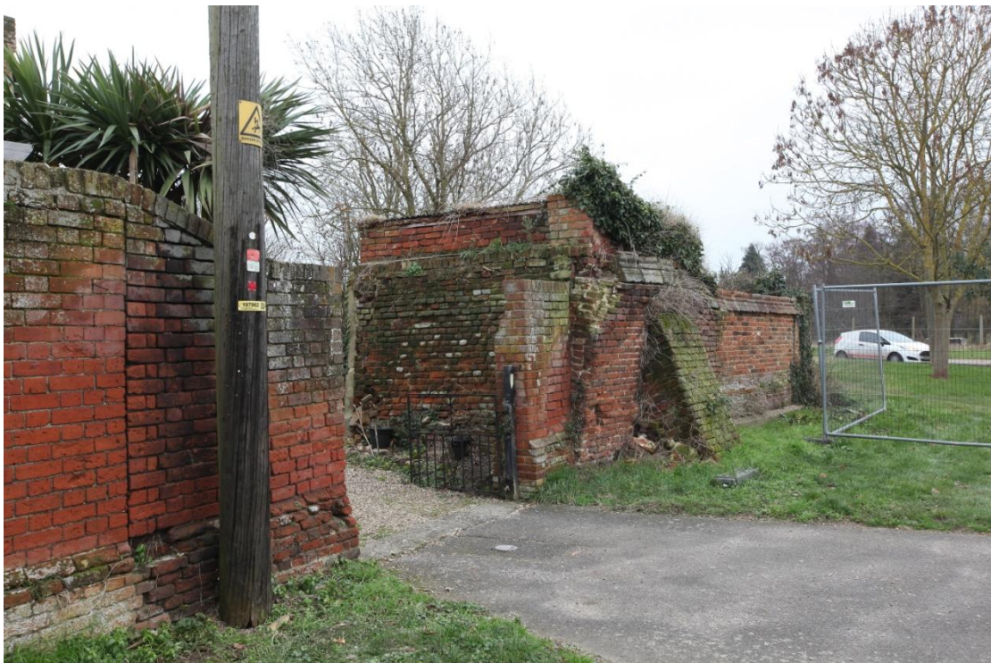
Illus. 28. The roadside wall from the north showing the vertical joint between the yard wall and the matching remains of the post-1839 pantiled farm shed to the left.
