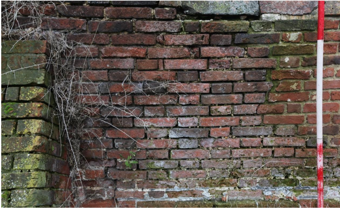
Illus. 13. Section 2 between the buttress (3) and the reconstruction (5) consists of narrow bricks laid in regular Flemish Bond in contrast to the irregular section to the left of the buttress (1). Uniform Flemish Bonding can be found in the 17 th century but is more usual in the 18 th and early-19 th centuries when this section was probably rebuilt.
