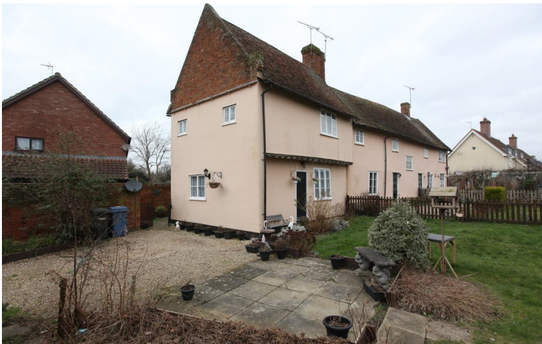
Illus. 4. The house from the south-west showing the slightly different axis of the two-bay jettied range at no. 12. This may have resulted from a desire to enlarge the rear courtyard of a demolished principal house in the foreground. The boundary wall to the left survives from the mid-19 th century single-storied shed shown in figures 8-10 which served the animal yard on the site of the modern house beyond. It has been cut on the right to create the present rear access to the no. 12. The latter's 'eared' brick gable may have survived from the 17 th century but has been rebuilt in recent years.
