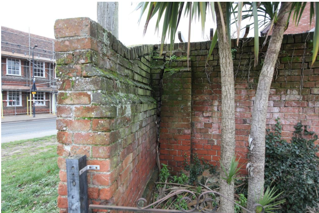
Illus. 26. The north-western internal corner of the garden belonging to no. 12 with the remnant of the pantiled mid-19 th century shed to the right and the contemporary or broadly contemporary section of roadside wall to the left. Both consist of uniform soft reds laid in Monk Bond with two stretchers between each header.
