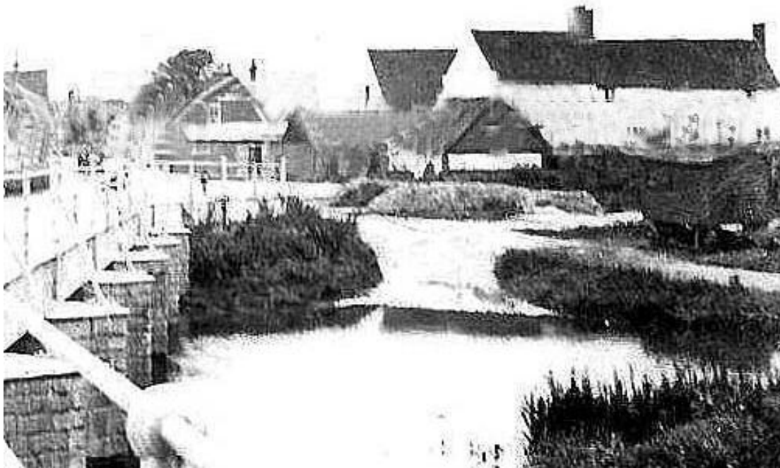
Figure 9. A similar early-20 th century view to that in figure 8, showing the house to the right with the large demolished barn in the rear. A mobile shepherd's hut lies on the waste ground to the right and the house is partly obscured by the detached shed that appeared against the wall between 1839 and 1884. This shed has also been demolished.
