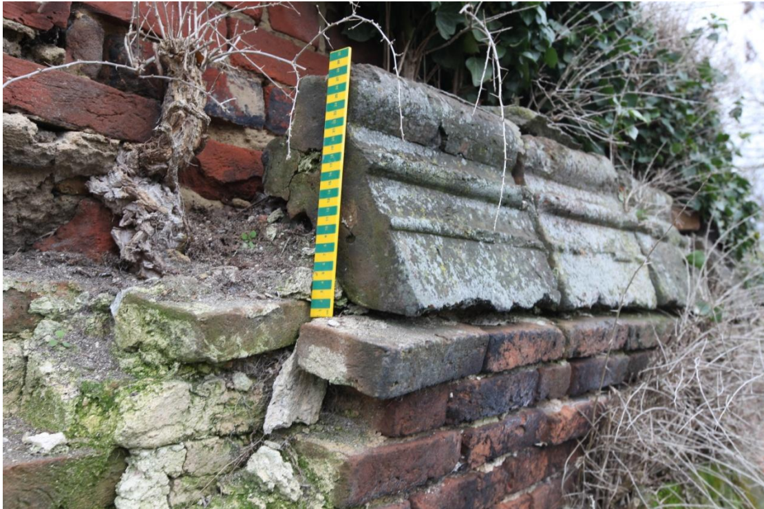
Illus. 19. A detail of the impressive coping tiles in illustration 18 which contain triangular frogs and side ridges of two different sizes below the roll of the ridge. The damaging new brickwork of the 20 th century shed (7) is visible at top left. The presence of a root has compounded the problem.
