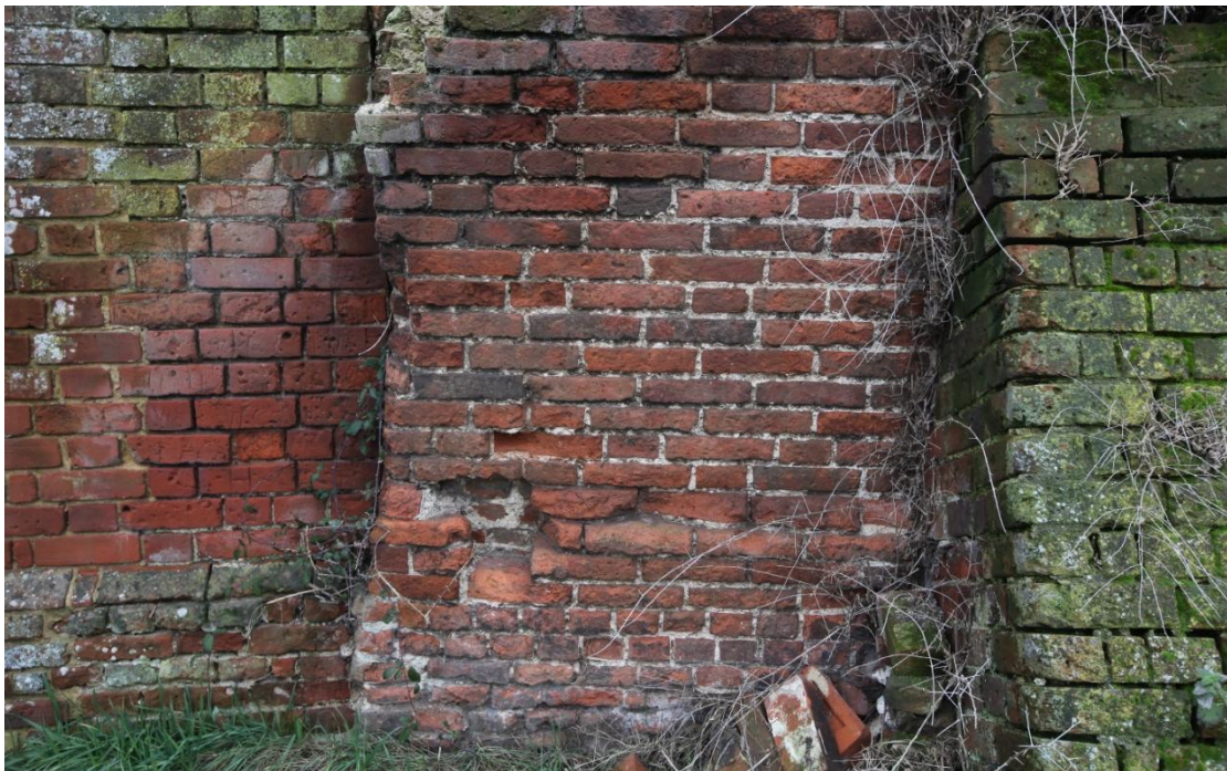
Illus. 14. The section to the left of the buttress in illustration 12 (1) is the oldest part of the structure and differs significantly from its counterpart to the right (2). Its narrow bricks of 9.25 inches by 2 (23.5 cm by 5) are laid in an irregular bond consisting of two or three courses of stretchers divided by courses of alternating headers and stretchers. The plinth is formed chiefly of headers. Brickwork of this kind is typical of the late-16 th and 17 th centuries, and may be contemporary with the jettied range of the house (i.e. no. 12). It has been truncated on the left where the corner consists of broken bricks, and the buttress presumably supports a hidden vertical joint against the rebuilt section (2).
