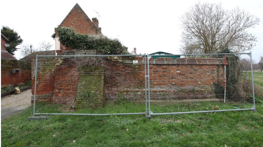
Illus. 8. The garden wall of no. 12 seen from Bridge Street to the south-west. The lower section to the right is lighter in colour and represents a recent reconstruction using old bricks on an earlier plinth but retains the impressive original coping tiles. It terminates in a new pilaster to the right but once continued further as shown on the historic maps. The section to the right of the 19 th century buttress is laid in Flemish Bond and is likely to date from the 18 th century while the section to the left is more random and may date from as early as the 16 th century. The short section adjoining the entrance to the extreme left was rebuilt in the mid-19 th century and matches its Monk Bond counterpart to the north of the entrance.
