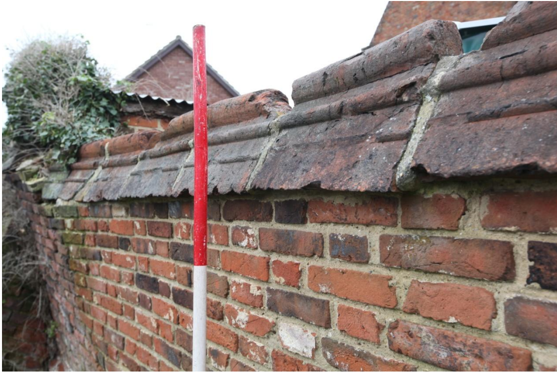
Illus. 11. A detail of the coping tiles in illustration 10 showing their two horizontal ribs of different sizes (6 in figure 12). These impressive features are difficult to date closely but may be as early as the 16 th century and are unlikely to be any later than the 17 th .
