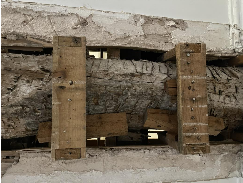
Fig. 11: Exposed timber beam underside
