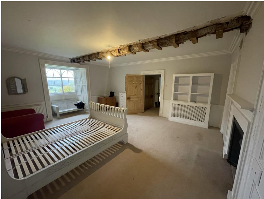
Fig. 12: Exposed timber beam first floor
