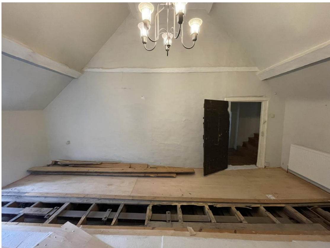
Fig. 7: Second floor with exposed beam
