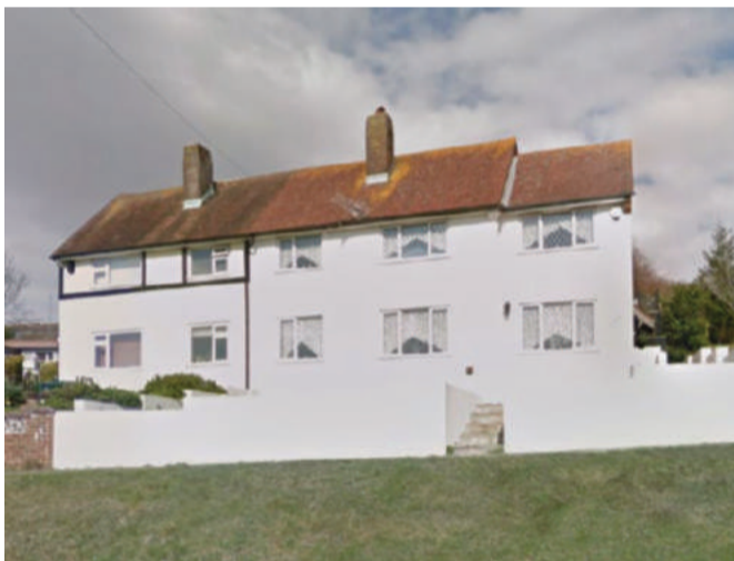
Example of two-storey side extension on Kenilworth Close
