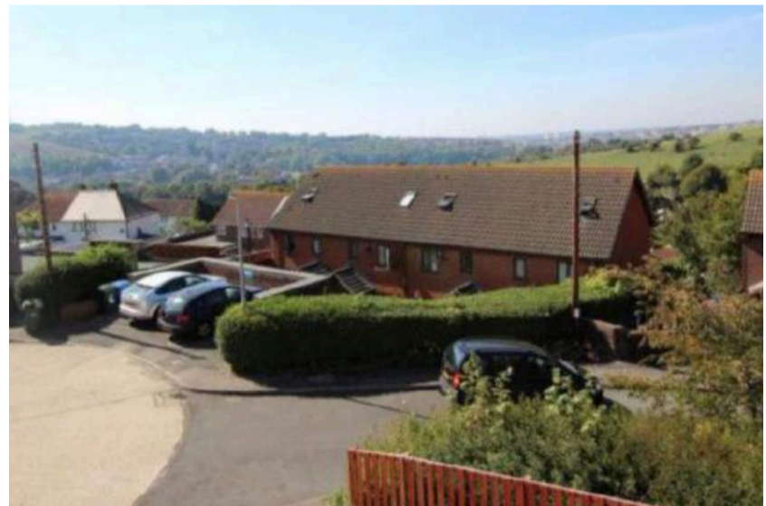
View from driveway accrossKenilworth Closelooking back toward Brighton
