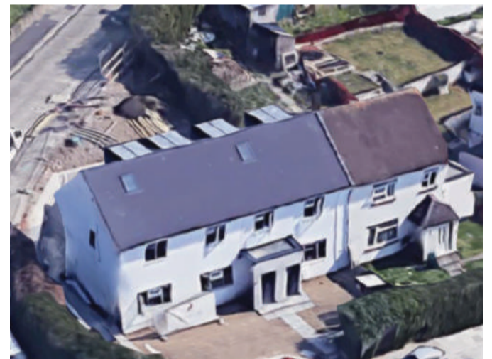
Example of significant side and rear extensions to split one dwelling up into multiple units - Norwich Drive. The proposal is extremely similar to the proposal at 24 Kenilworth Close.
