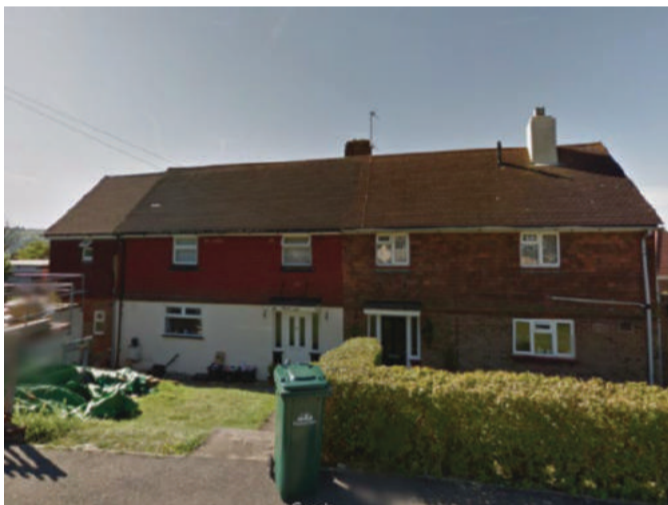
Example of two-storey side extension on Kenilworth Close
