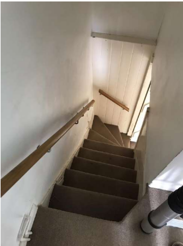
View down the stairs to no.9 from the first floor landing.
