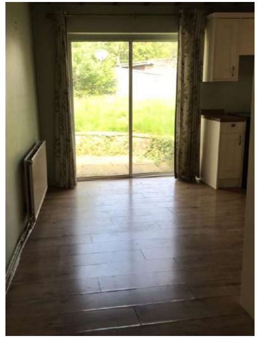
Right - Internal view of the kitchen extension looking towards the patio doors from the opening in the rear of no.7
