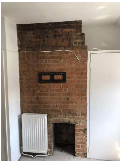
Left – view of the original chimney stack to the first floor room to no.7 and small open fireplace, with a cupboard to the right.
