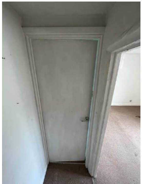
Right – view of the door from within the small landing
