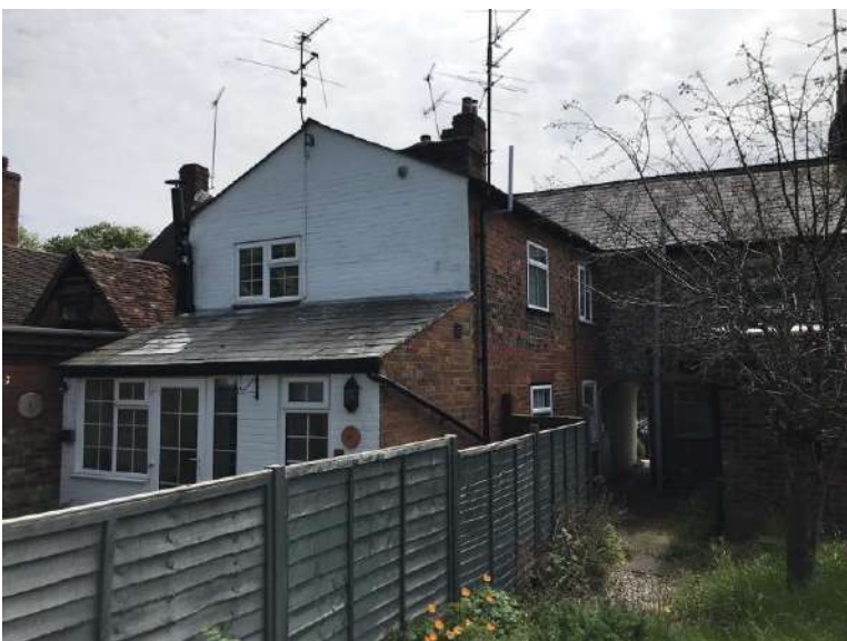
View from the rear garden towards the back of no.11, showing the garden fence and rear single storey element to no.11 and the two storey element with its combination of facing brickwork, painted brickwork and slate roof.
