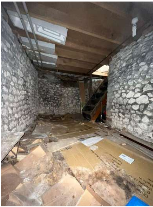
Left – view of the cellar looking towards the staircase
