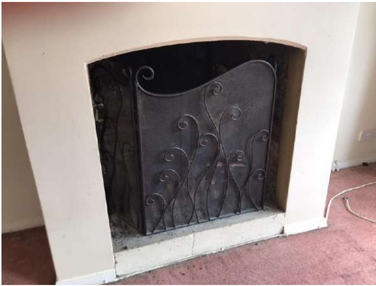
View of the ground floor fireplace to no.7, showing no mantel piece of decorative grate.
