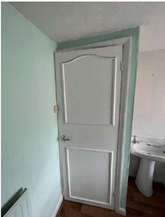
Left – view of the door from within the bathroom
