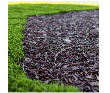
Footpath Resin Bound Rubber Mulch Surfacing
