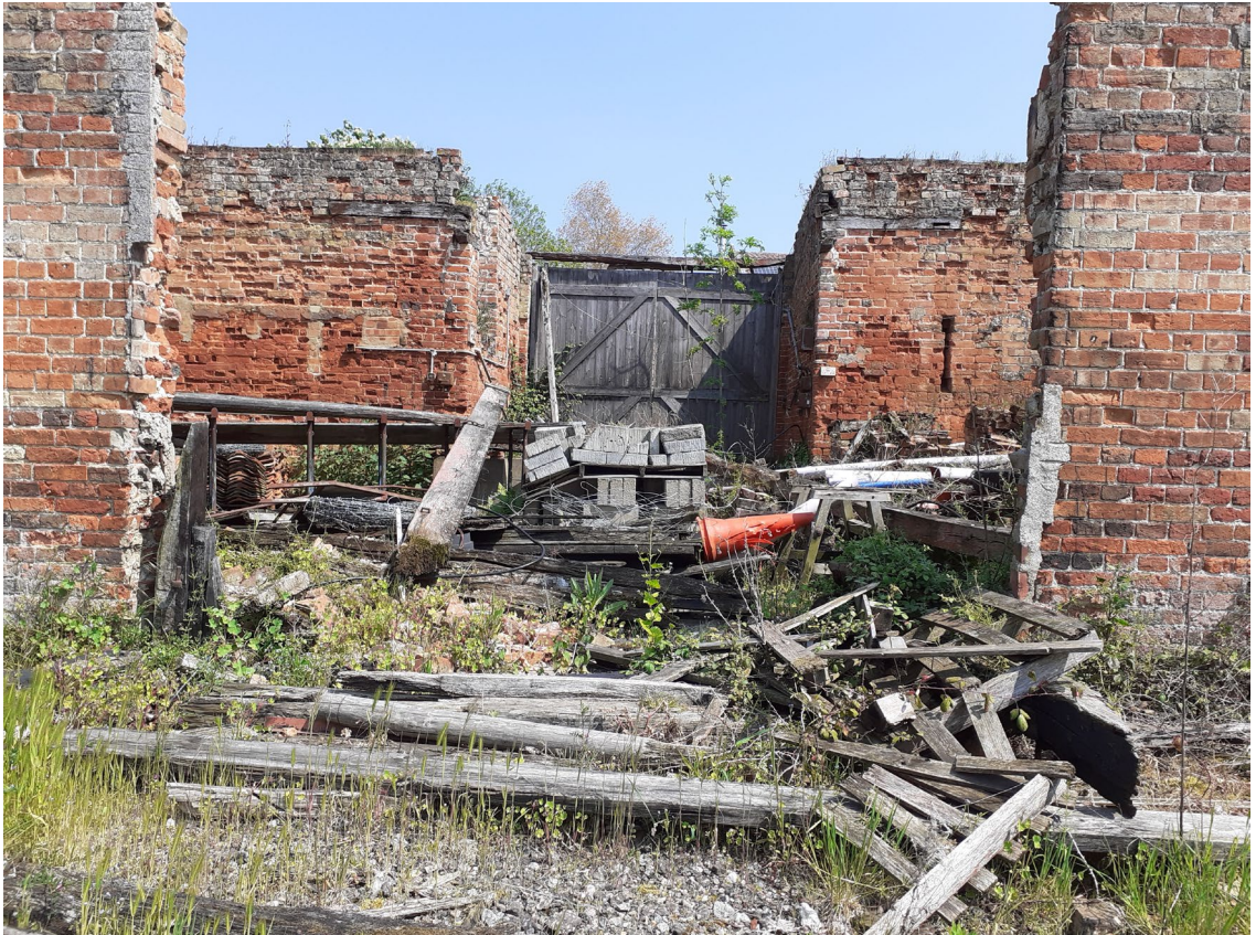
Photograph 5: Building materials and debris internally
