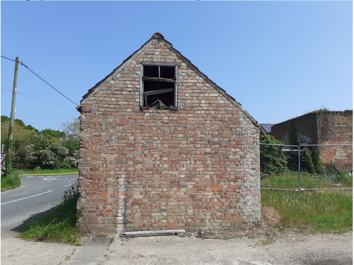
Photograph 10: External western elevation.
