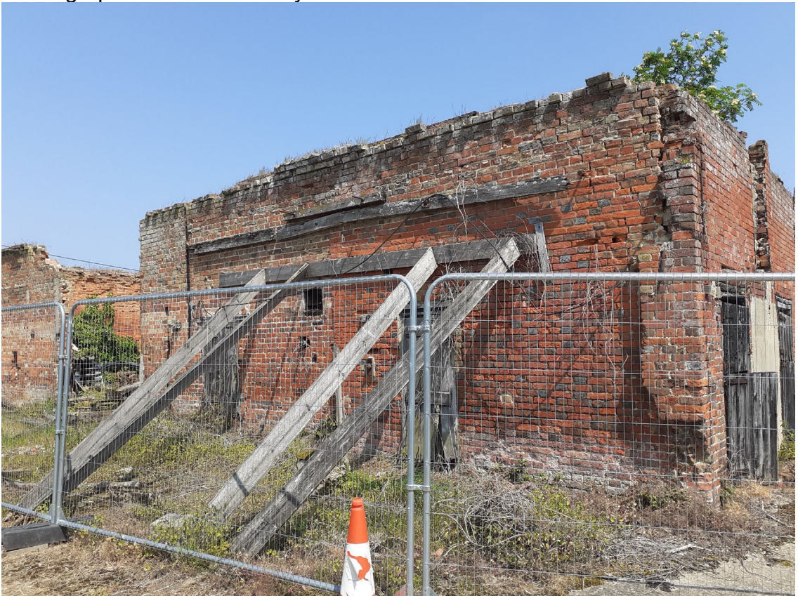
Photograph 4 : View of the south-western propped external wall.
