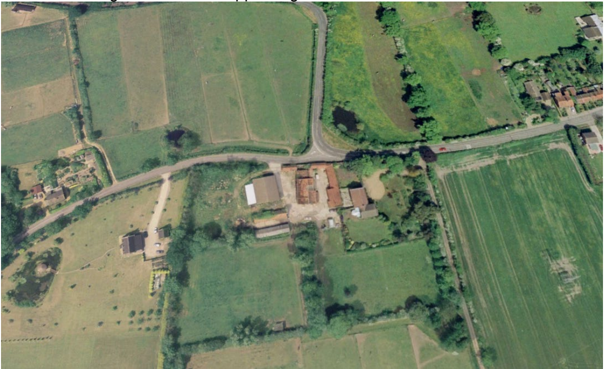
2006 aerial image shows the deterioration to the structure.
