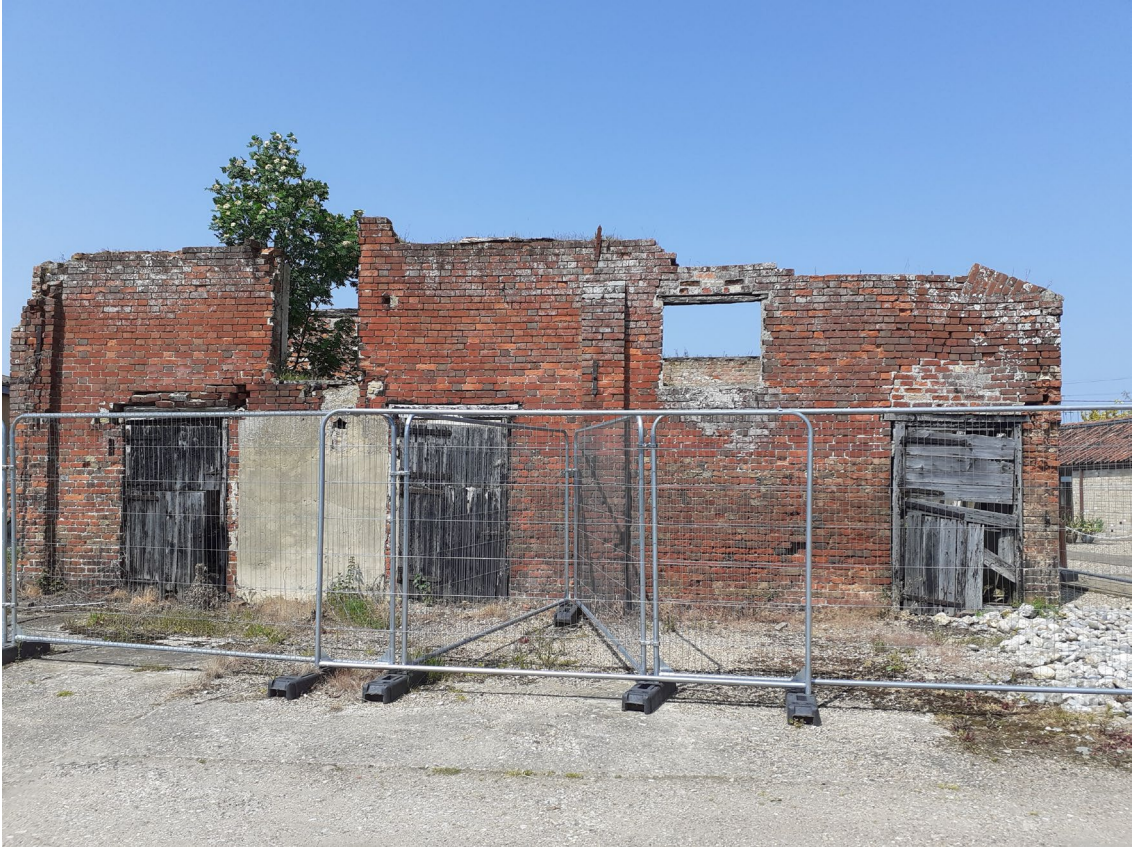
Photograph 1: Southern elevation of main barn.
