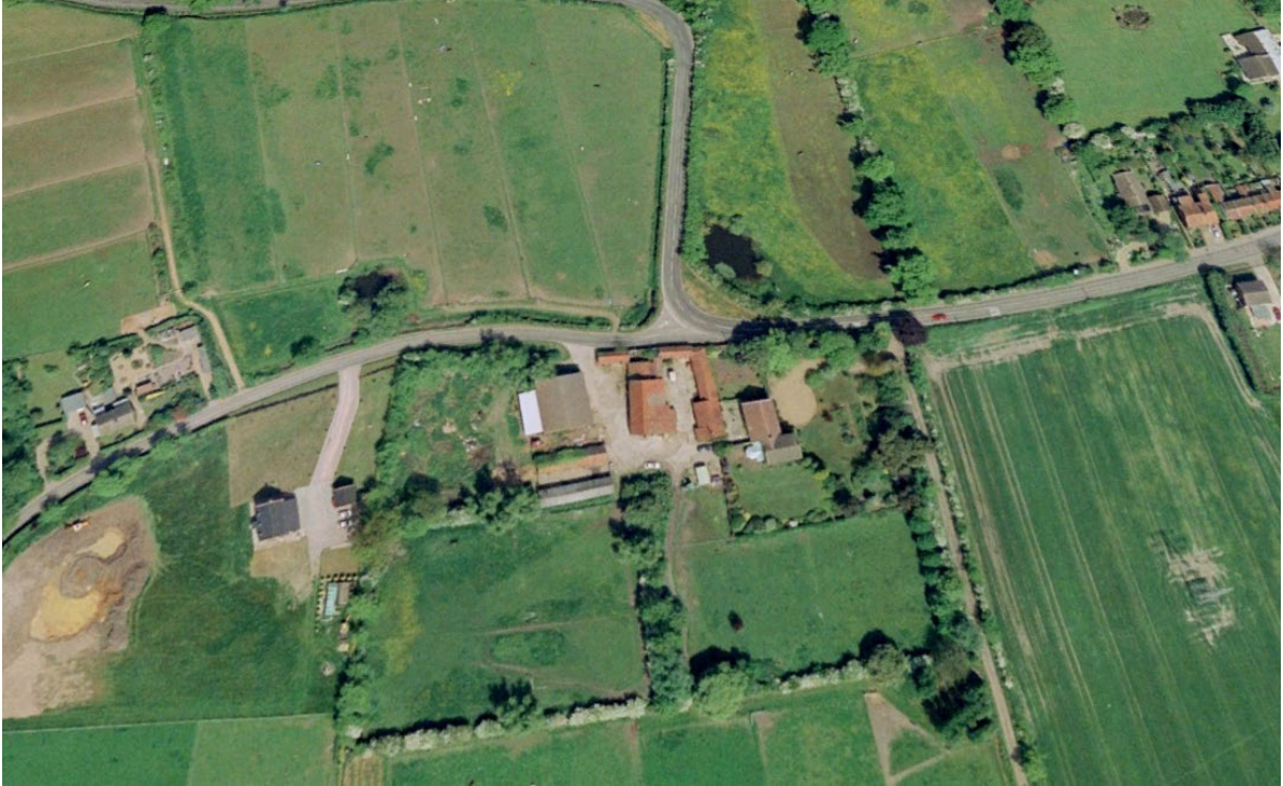
1999 aerial image with the roof appearing in a sound condition.
