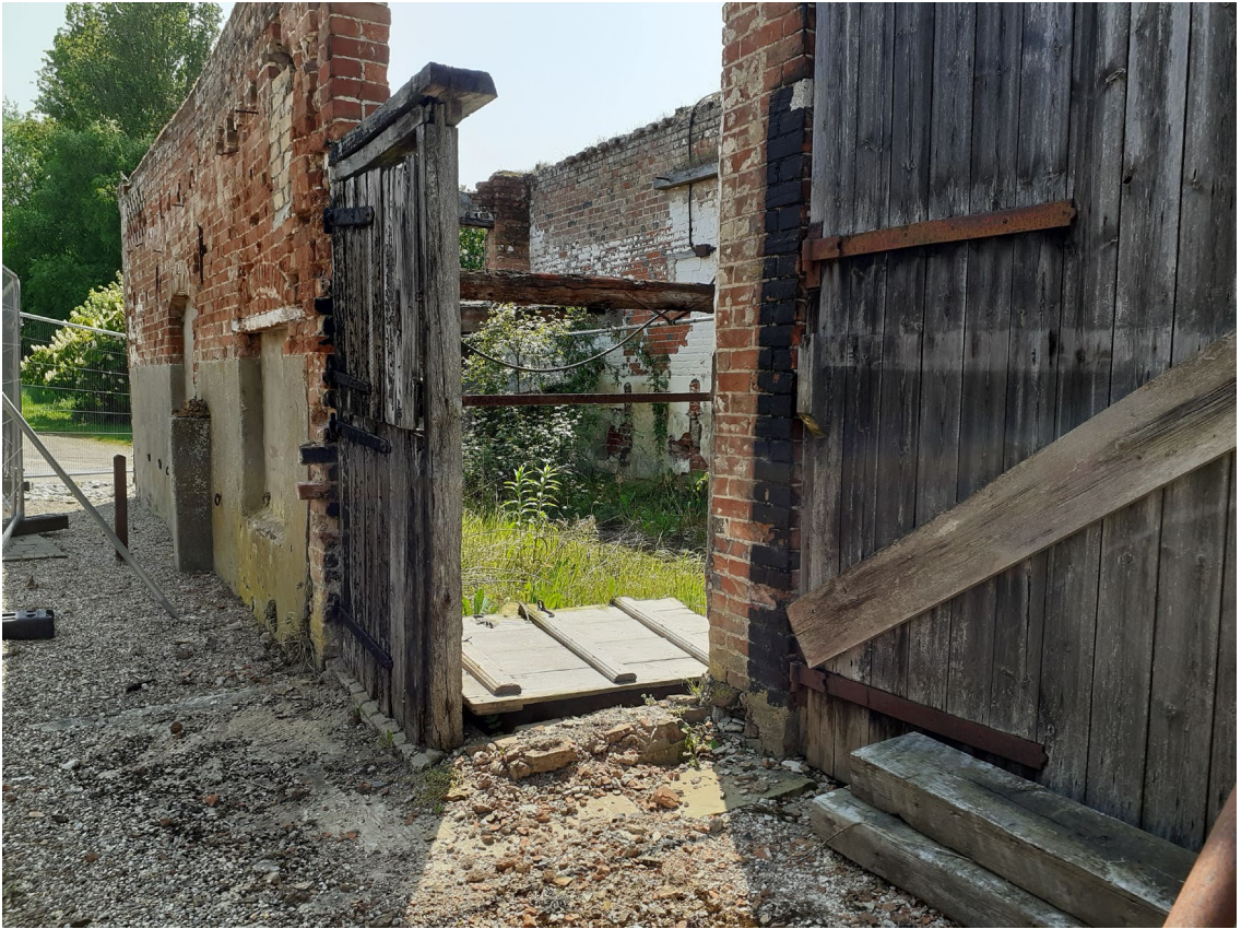
Photograph 3 : View internally on the eastern side.
