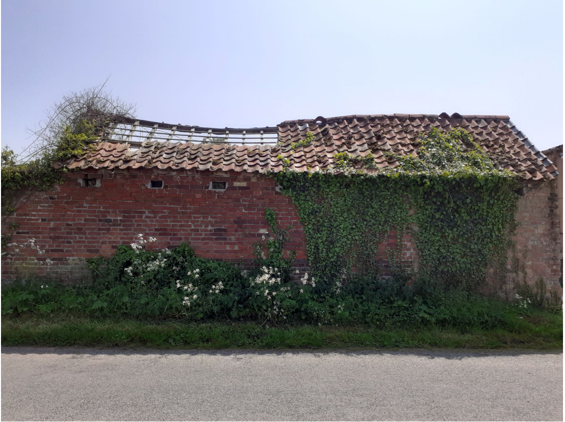
Photograph 9: External northern elevation adjacent to Hall Lane.
