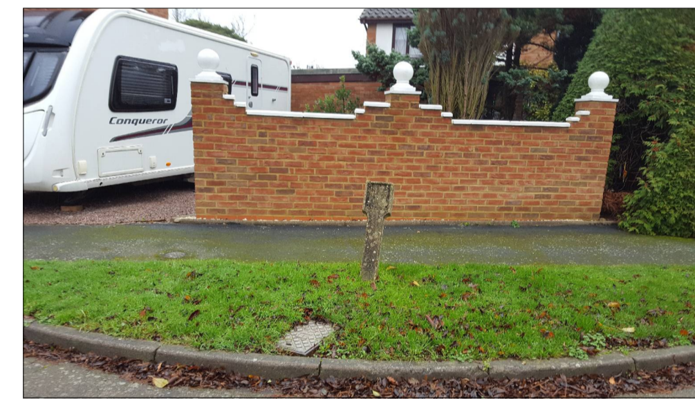
FIG. 1 - NEW WALL REPLACING HEDGE
