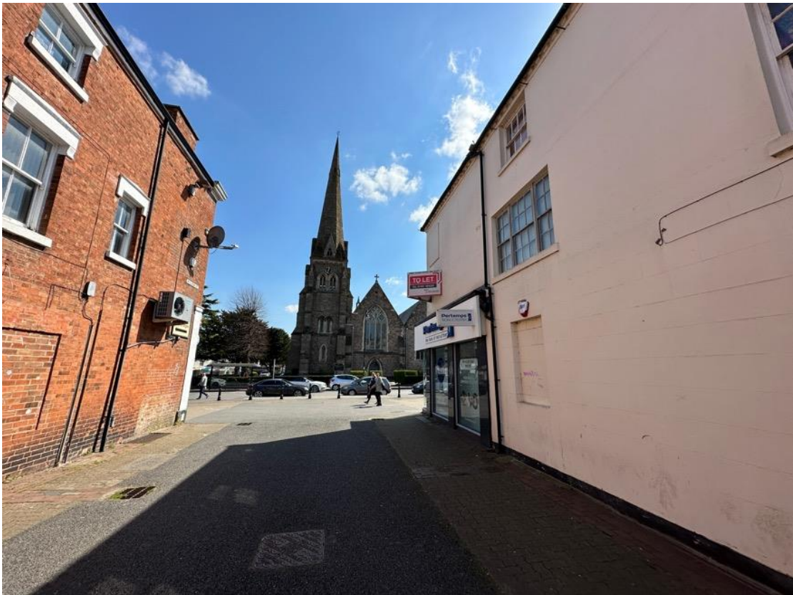
Figure 32 No.6 frames one side of the view from William Street towards St Stephen's Church.
