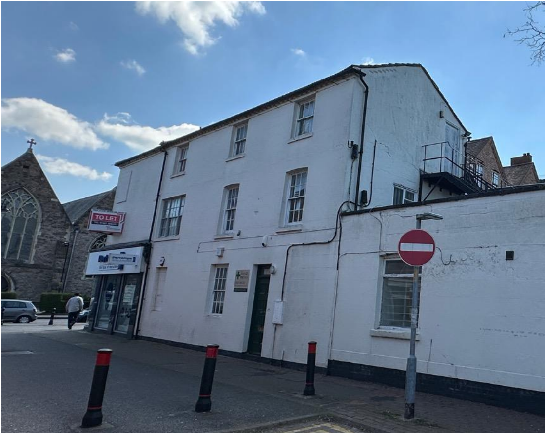
Figure 8 Three storey 3 bay property (centre) fronting onto William Street.
