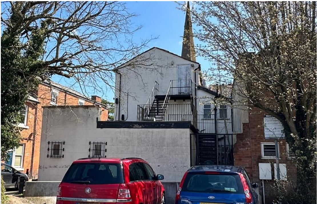
Figure 29 The west elevation off William Street which includes a fire escape onto the flat roof.
