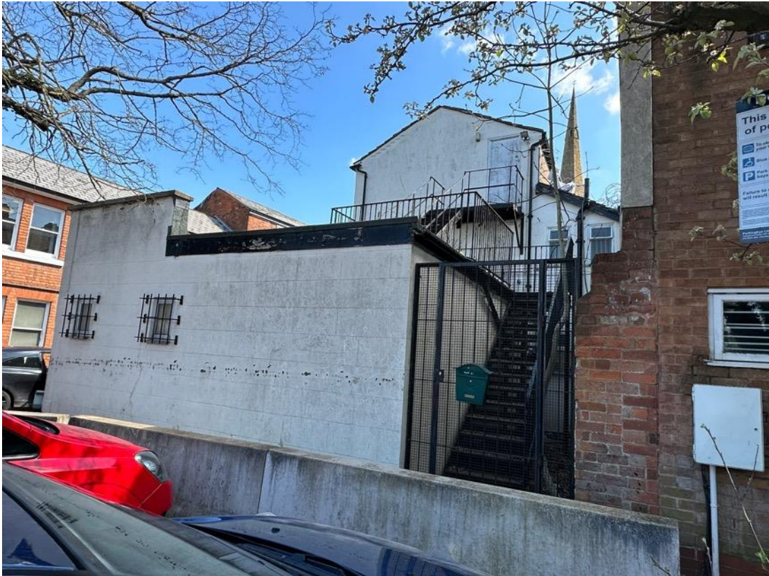
Figure 20 West end of the application site showing 20th century extension.
