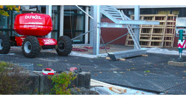
TuffTrak® ST is the ultimate standard heavy duty road mat ideal for use as temporary roadways, work areas for heavy plant and machinery, drilling rigs, depot or storage areas.
