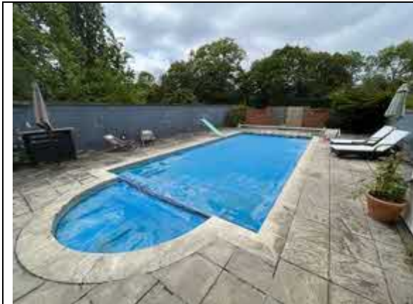
Photo 1. Swimming pool and surrounding paving
