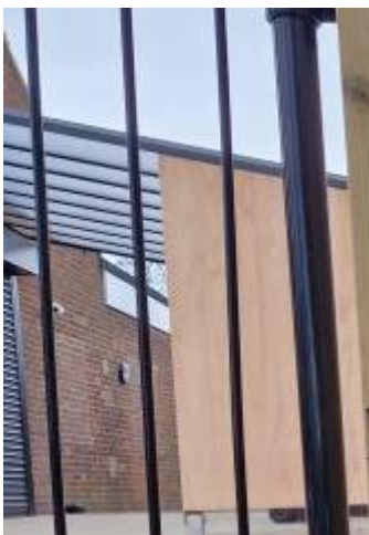
Existing side store and canopy
