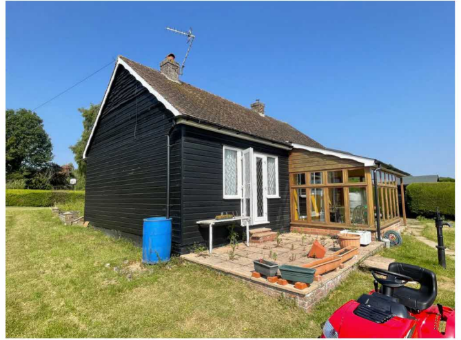
Photograph 2: Rear elevation of Dingley Dell
