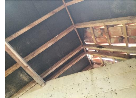
Photo 15: 3a – low internal wall.
