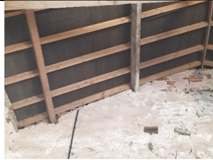
Photo 10: Internal gable wall.
