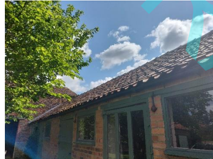
Photo 13: Roof of 3a & 3b.
