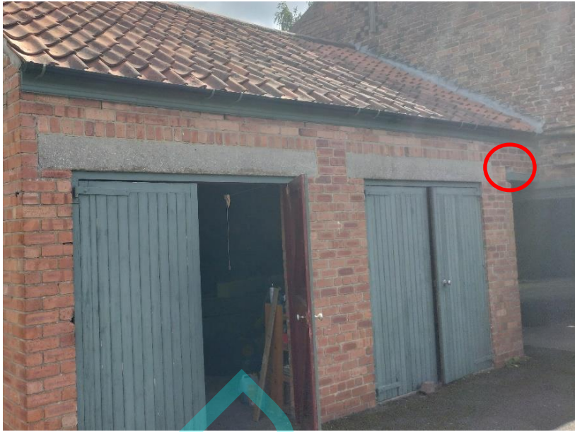
Figure 5. Emergence location 1; Building 1
