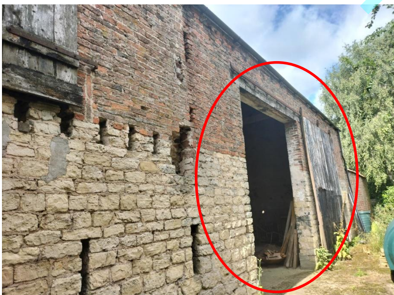
Figure 9. Emergence location 7; Building 2
