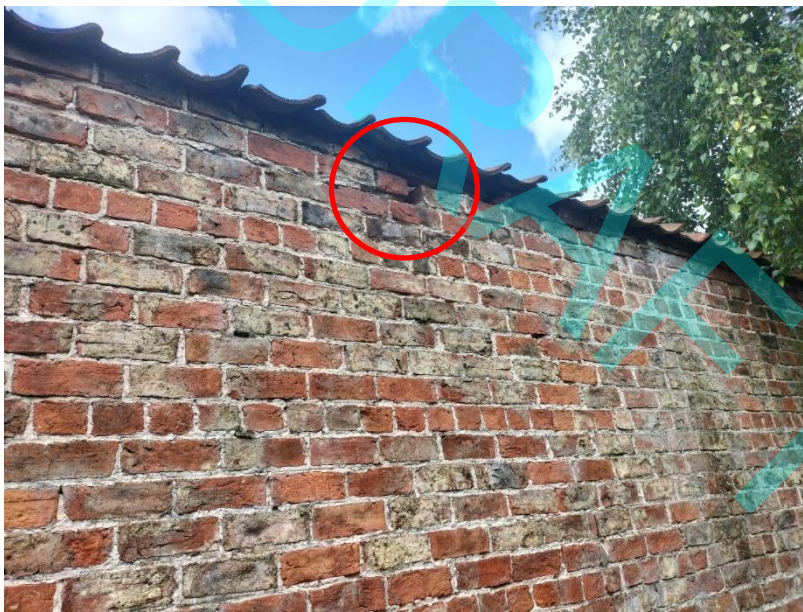
Figure 6. Emergence location 3; Building 1
