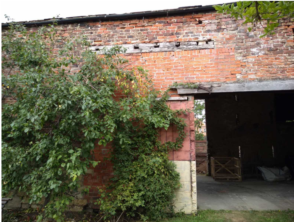
Photo 2 –Front Elevation Doorway alterations
