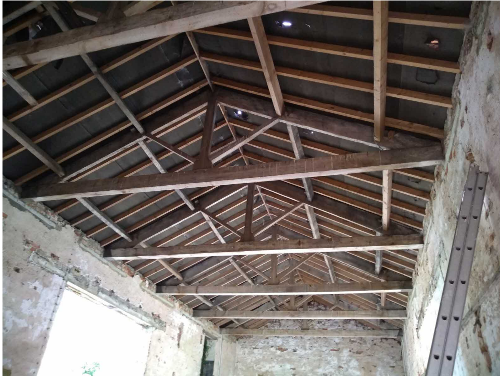
Photo 9 –King post roof trusses
