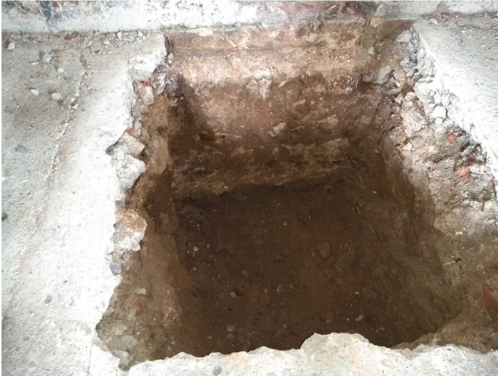
Photo 13 –Trial hole 4 right-hand gable
