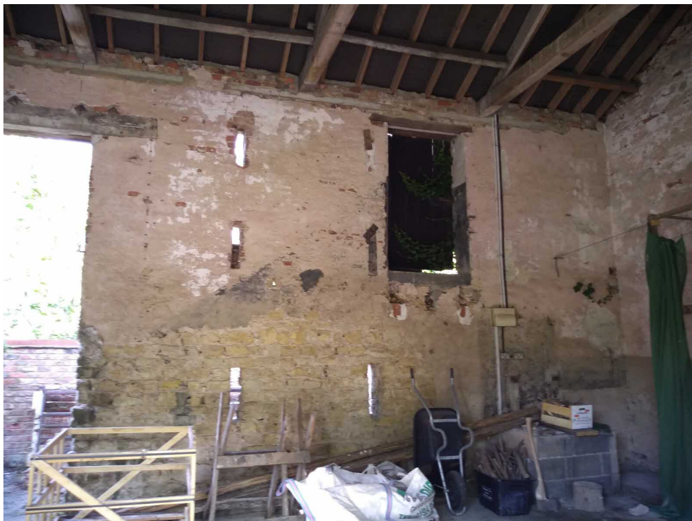
Photo 10 –Internal of rear elevation showing truss bearing
