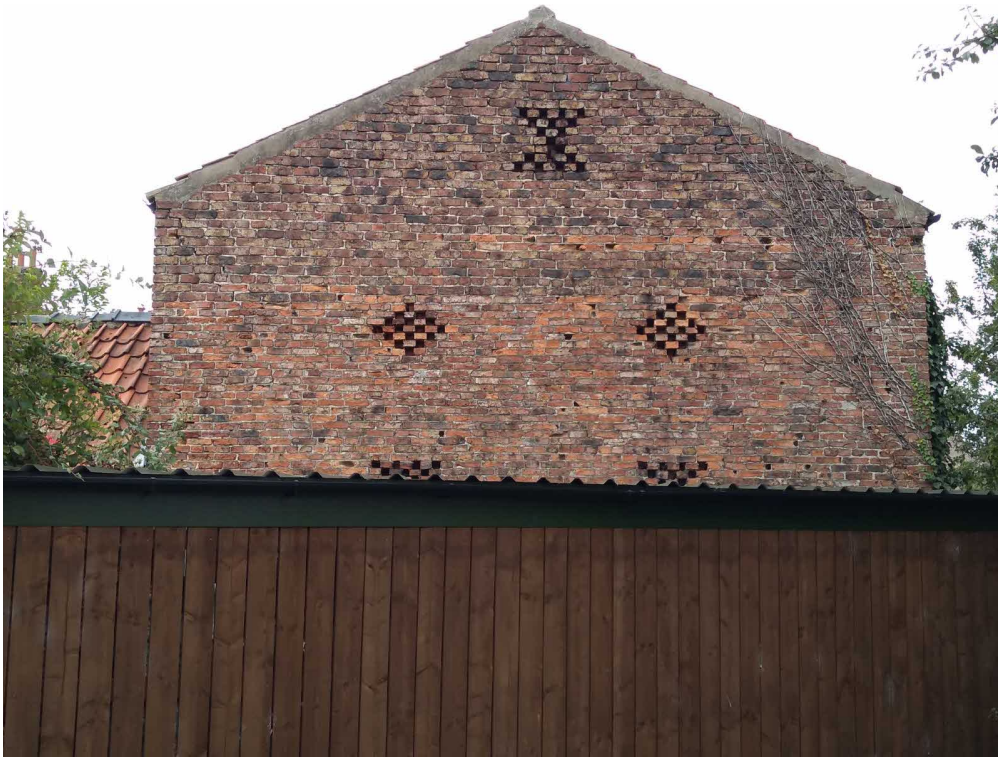
Photo 5 –Right-hand gable elevation
