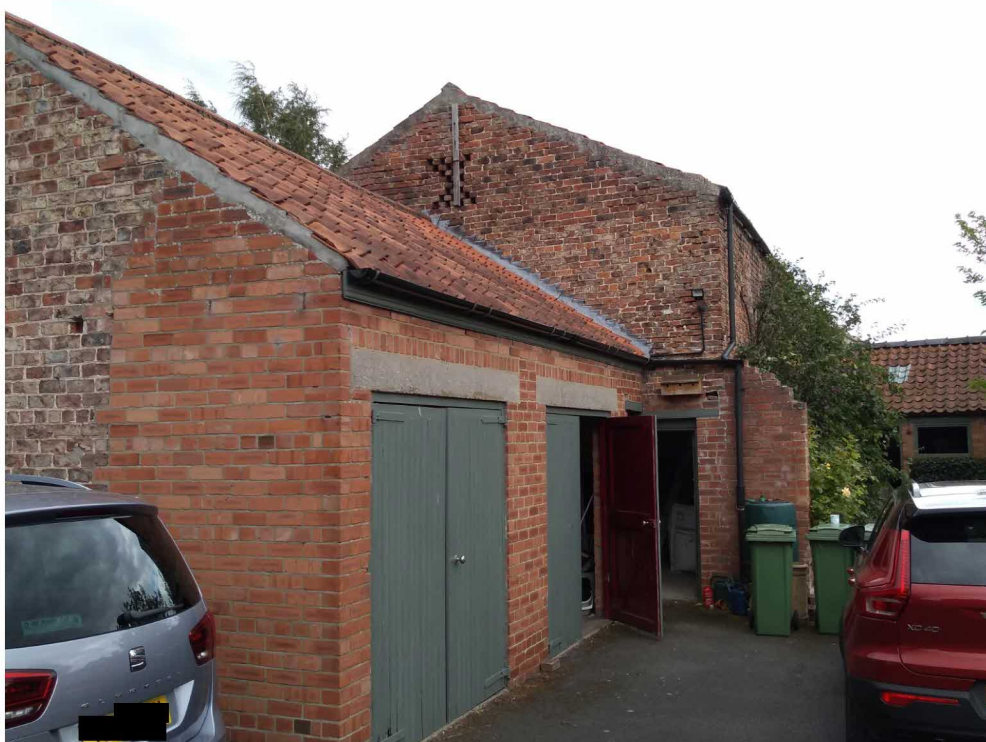
Photo 4 – Left-hand gable elevation
