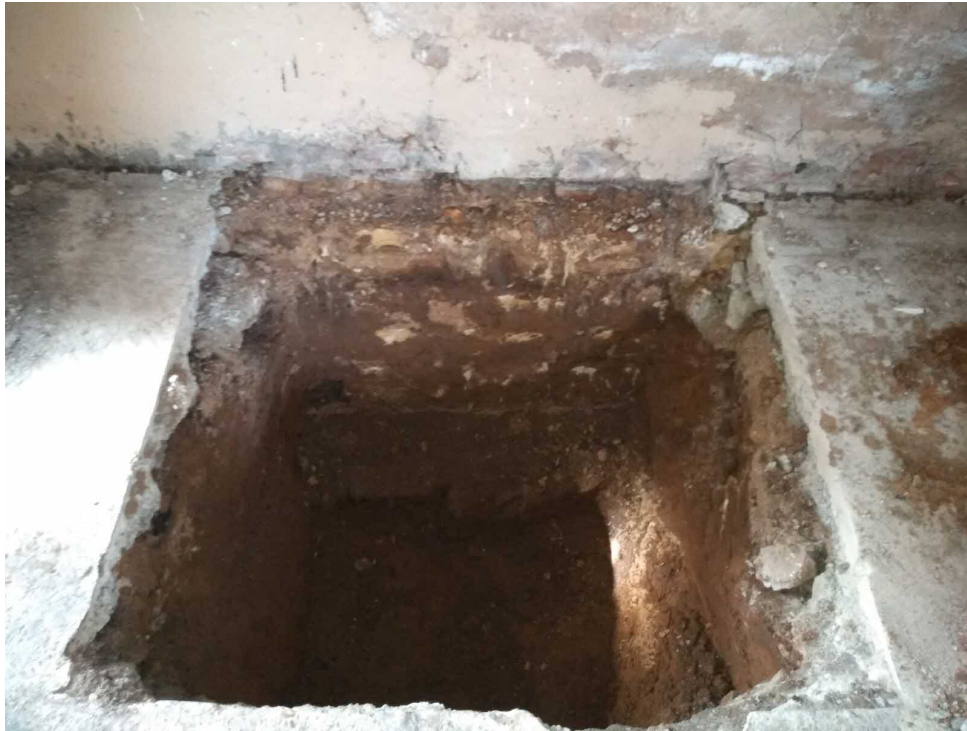
Photo 11 –Trial hole 3 left-hand gable
