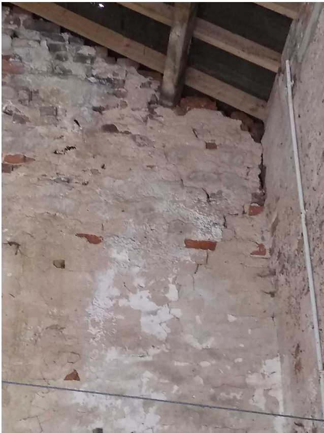
Photo 14 –Right-hand gable at high level
