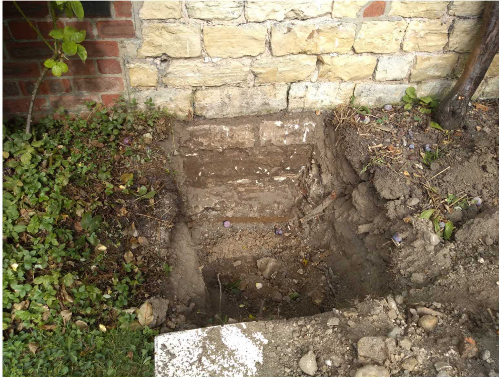
Photo 3 – Trial hole 1 Front elevation
