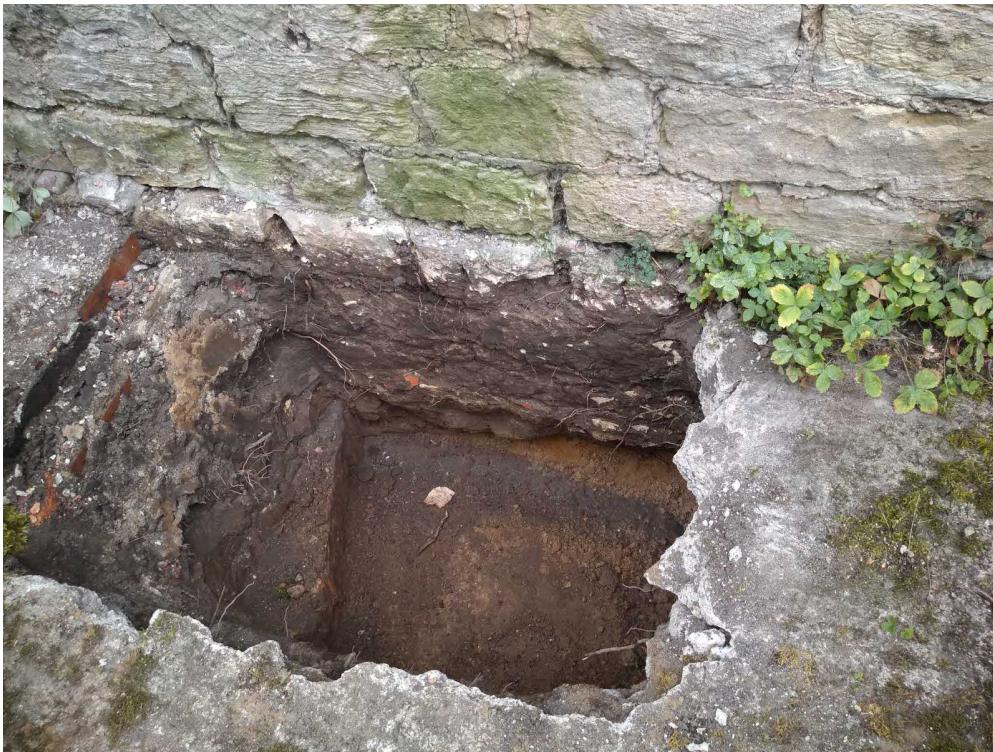
Photo 8 –Trial hole 2 rear elevation
