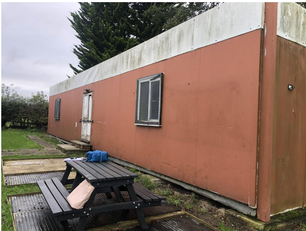
Photo 2: East elevation of the existing portacabin.
