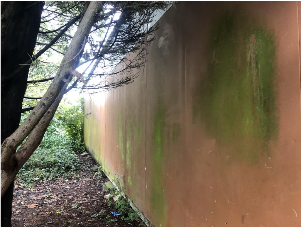
Photo 4: West elevation of the existing portacabin.
