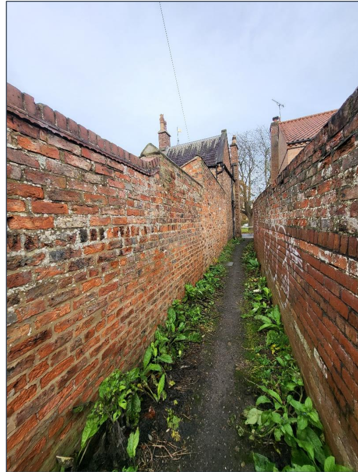
Figure 12 View north along Love Lane (No.16 on left, No.14 on right)
