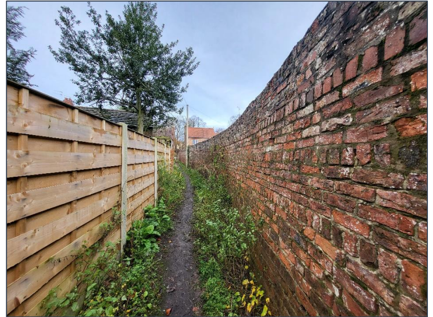
Figure 18 View north along Love Lane with leaning wall of the Site on right. Note change in brick to top third.
