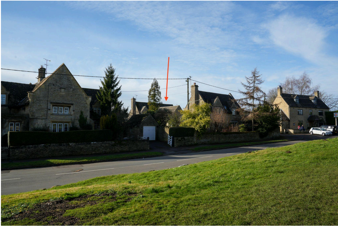
Obscured view of rear elevation from All Saints Church
