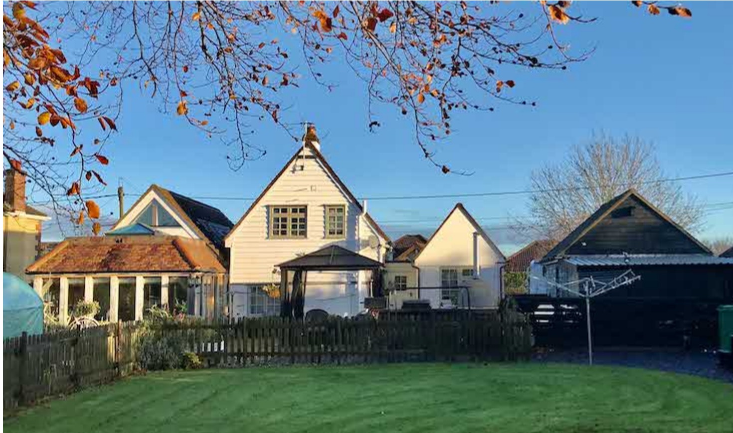
Above: rear elevation of Pear Tree Cottage. Five distinct volumes comprising (left to right) 1. Timber-framed orangery in front of 2. Pitched roof 1.5 storey extension with gable glazing; 3. Principal volume/main house white weatherboarding with pitched roof in plain clay tile; 4. Smaller single-storey pitched roof extension, white render and clay tiled roof, linked to main house, and 5. Black weatherboarded detached cartlodge with slated and pitched roof.
