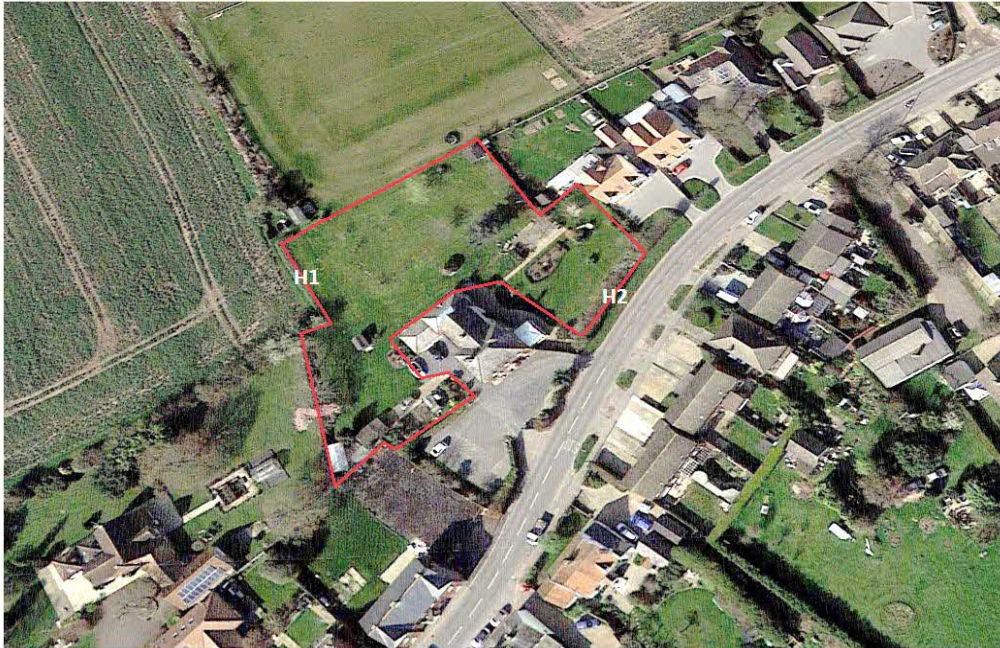
Fig 2. Aerial Site View and Buildings – Google Earth, March 2022
