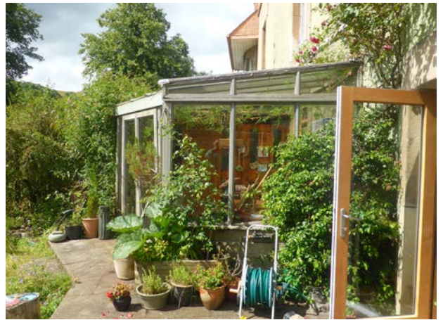
View to side of existing conservatory.
