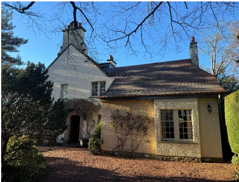
Extension to the East elevation was carried out and completed 1990 – 1991
