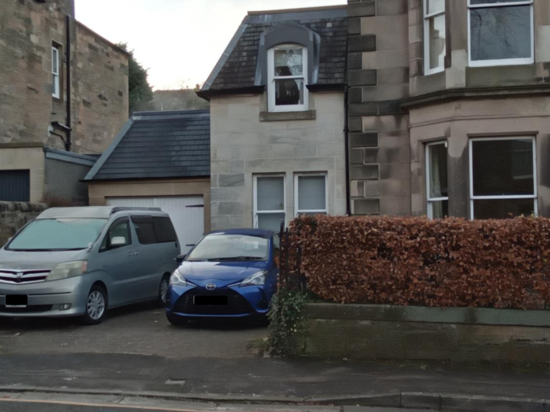
Examples of extensions, traditional and contemporary solely within Mansionhouse road.
