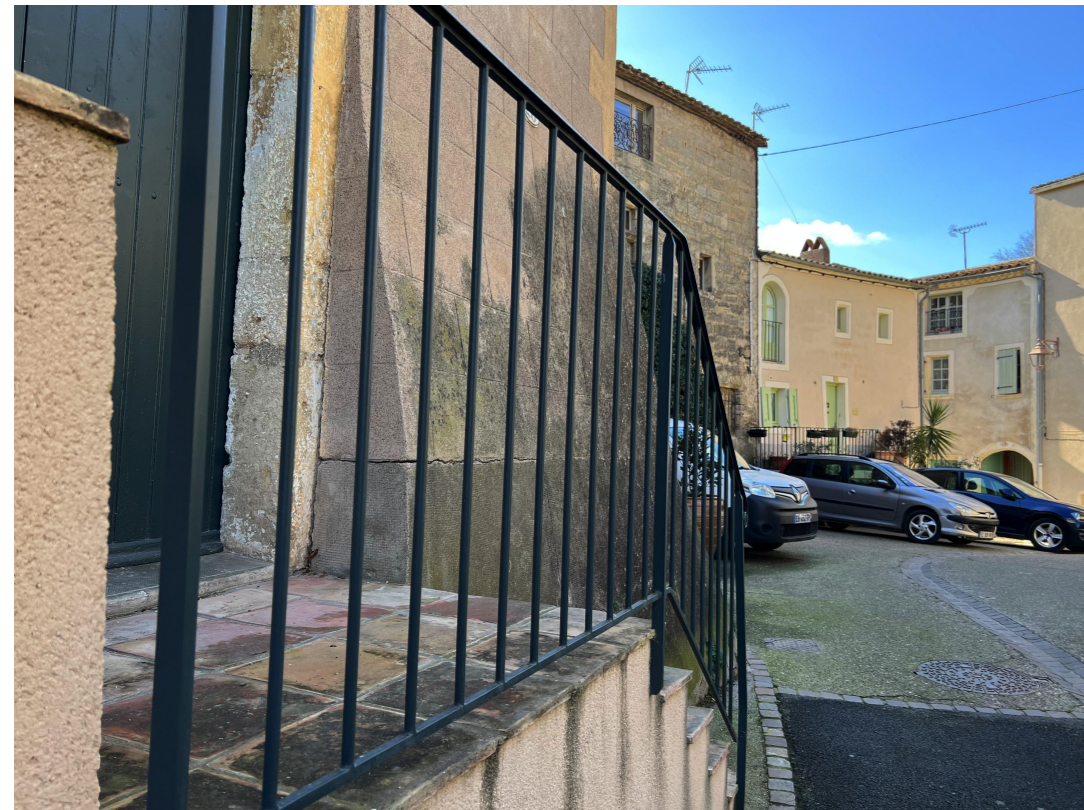
B - vertical metal railing
