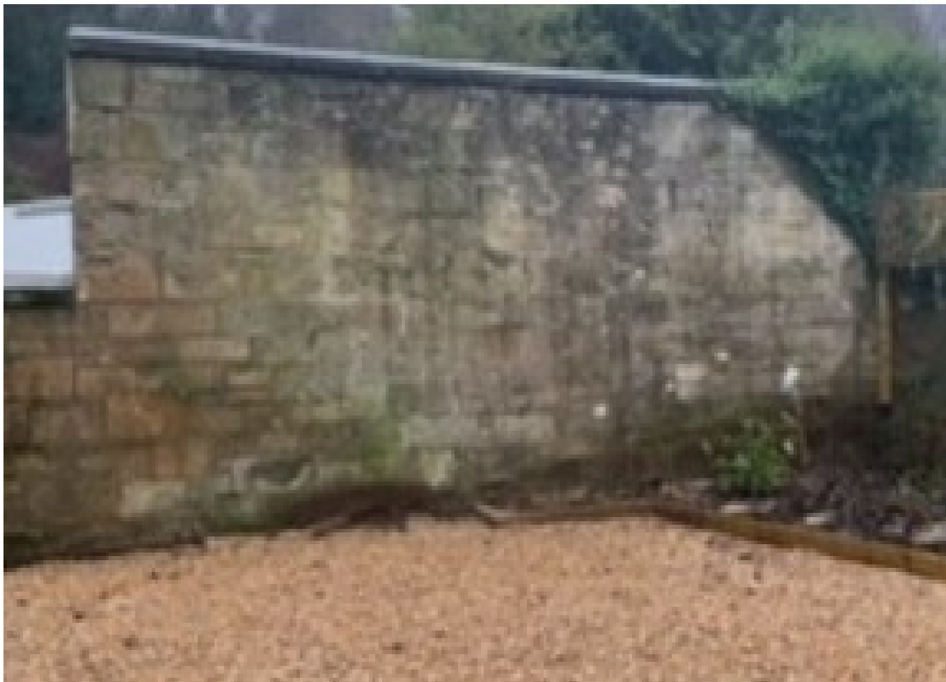
VIEW OF FRONT GARAGE WALL - NATURAL STONE
