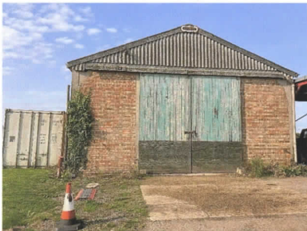
Photo 1: Eastern façade of Barn 1, with metal container adjacent to the south
