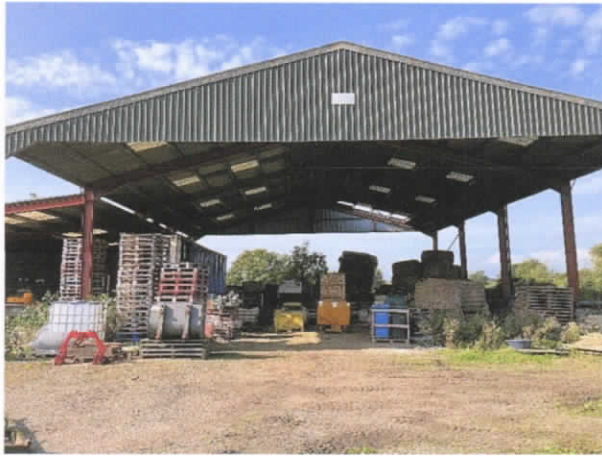
Photo 5: Barn 3 - eastern façade through to rear (western) façade
