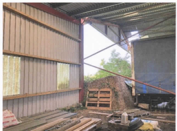
Photo 4: Internal view of Barn 2, with straw bale western rear wall of Barn 2 visible adjacent to metal sheet wall section
