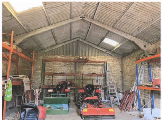
Photo 2: Internal view of Barn 1
