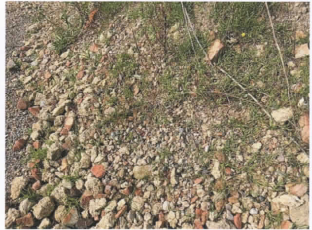
Photo 12: Northern eastern rubble pile – vast majority is fine and well consolidated, with some larger looser rubble at base
