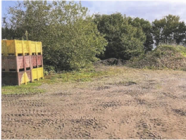
Photo 11: Hard standing, bare ground and compacted hard core in north eastern corner of site. Mature goat willow also present. Mature hazel in far eastern corner, adjacent to rubble pile
