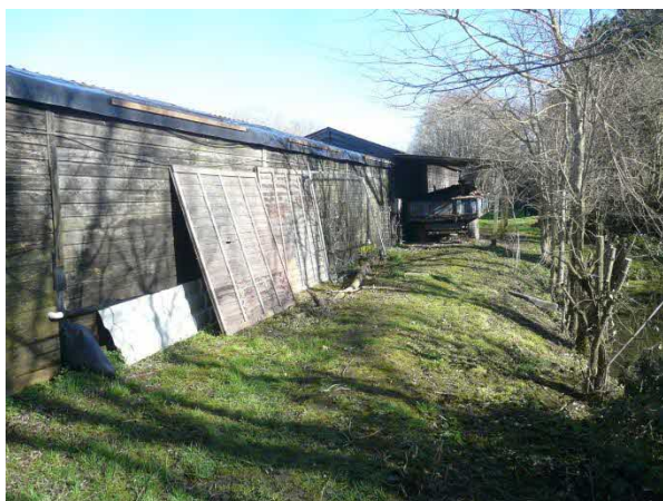
Plate 5: Southeast aspect of the stables.
