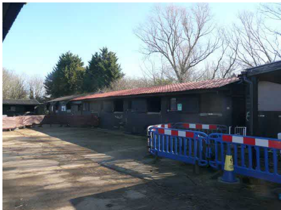
Plate 3: Southwest aspect of the stables to be developed.
