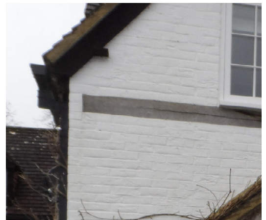
Painted Brickwork As ex Cottage
