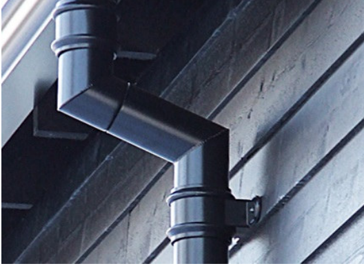
Black metal rainwater pipes
