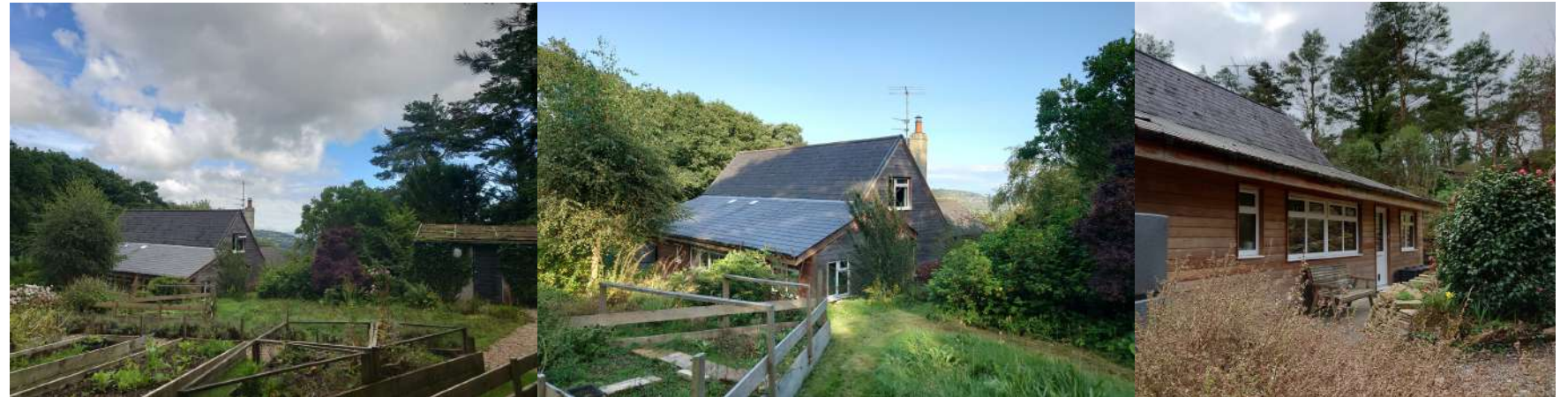
Figure 3. – View of existing house from Seaview Road
