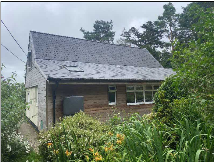
Photograph 3: Exterior viewed from the northeast
