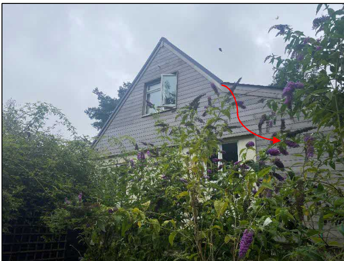
Photograph 8: Emergence point of bats on the northeast gable end on 15.08.23
