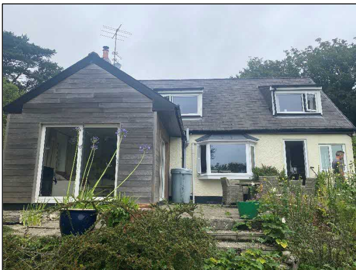
Photograph 1: Exterior viewed from south-west
