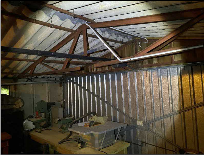
Photograph 6: Internal of garage
