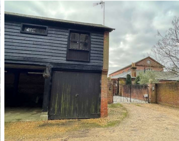
Figure 29 – Access to the courtyard to the side of No 4 with barn in distance
