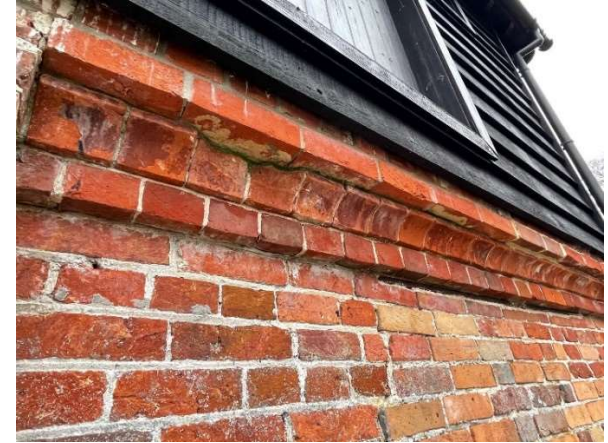
Figure 20 – Staggered central brick detailing to rear
