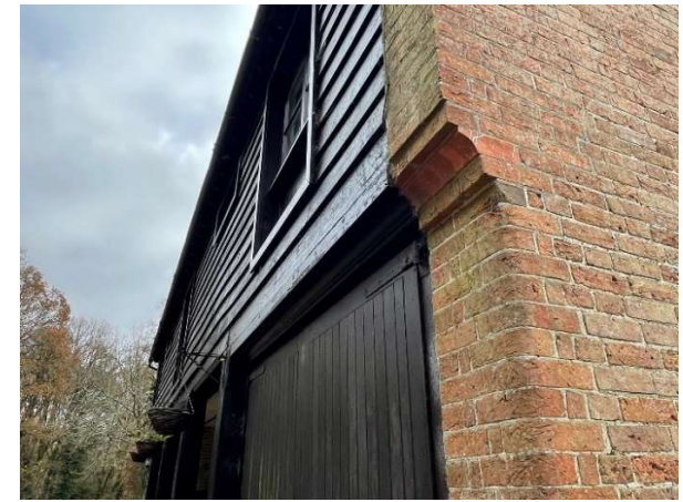
Figure 17 – Brickwork detail to corner including curved bricks
