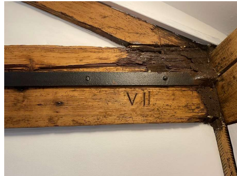
Figure 34 - Carpenter Marks
