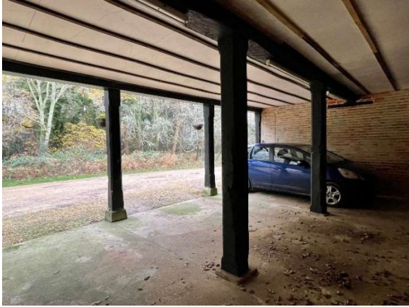
Figure 18 – Within the cart shed
