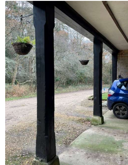
Figure 23 – Openings between timber posts
