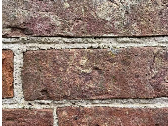
Figure 19 – Penny struck pointing
