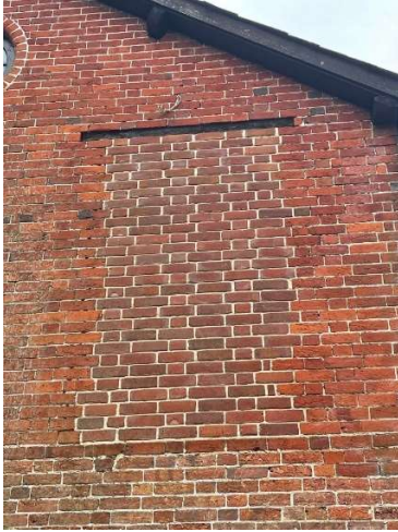
Figure 24 – Blocked doorway opening to western elevation at first floor
