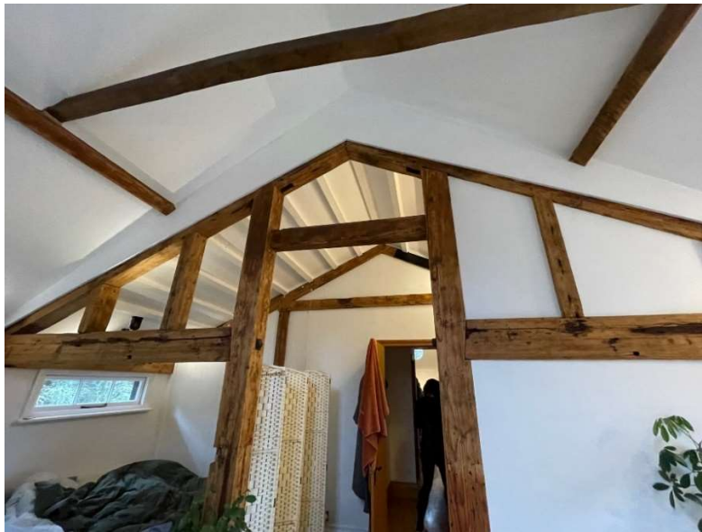
Figure 33 – Internal trusses, showing partial infilling
