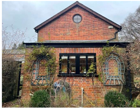
Figure 16 – Eastern side elevation, with late 20 th century lean-to extension (also a bullseye window)
