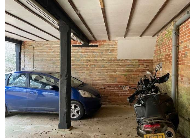
Figure 26 – Internal space under first floor looking east
