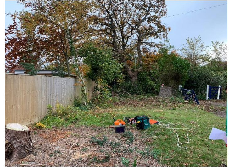
Photo 9: North area of the site
