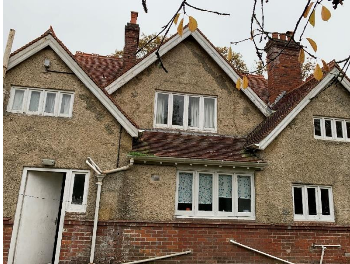
Photo 2: West elevation of dwelling
