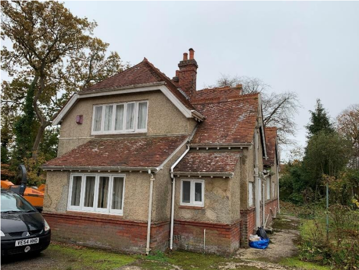
Photo 1: North elevation of dwelling
