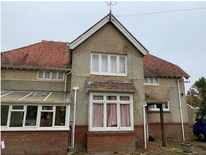
Photo 4: East elevation of dwelling
