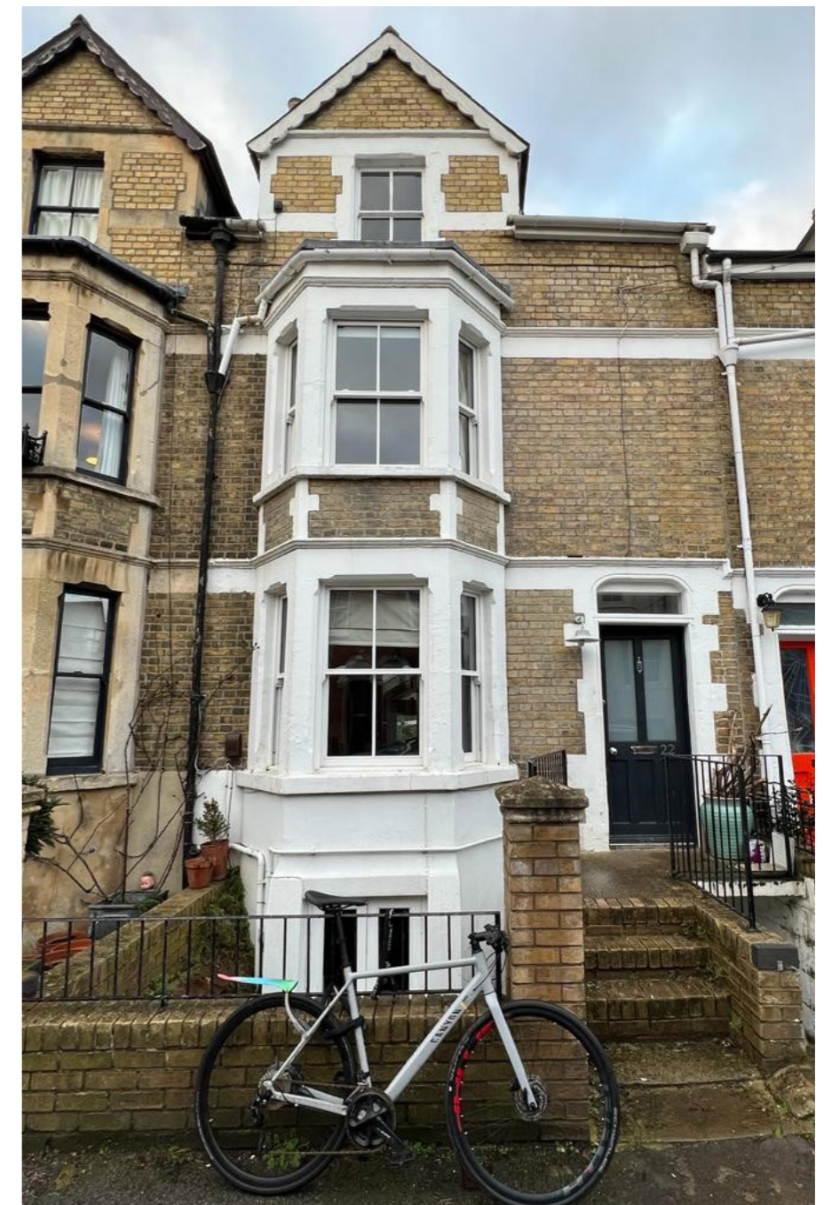
Existing Front View
