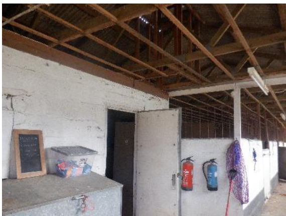
15. Breezblock walls and stables within the building, internally open to the roof (B2).
