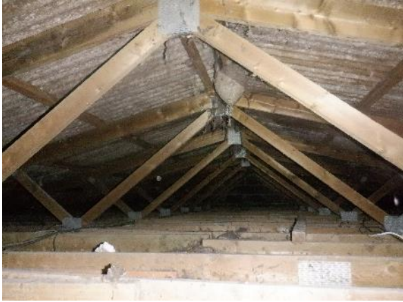
31. Heavily cobwebbed ridge and un-boarded floor within the roof void (B6).
