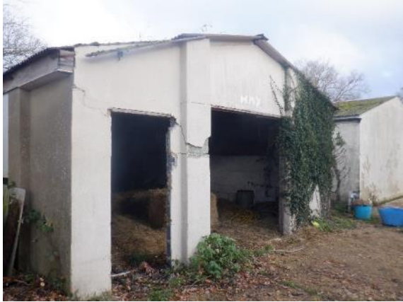
19. Small storage barn viewed from the south (B5).
