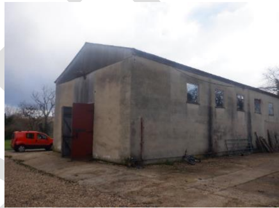
10. Large storage building viewed from the north-west (B1).
