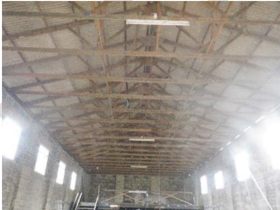
11. Internally open to the ceiling with the underside of corrugated sheets visible (B1).
