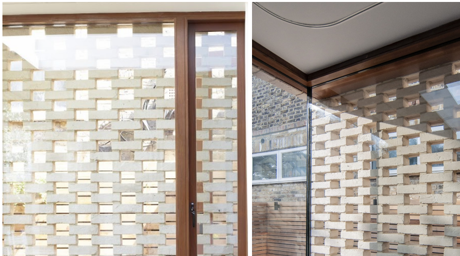
Fig 4.2 - Precedent images of 'hit+miss' brick screen. Creating security and privacy while allowing light to filter through
